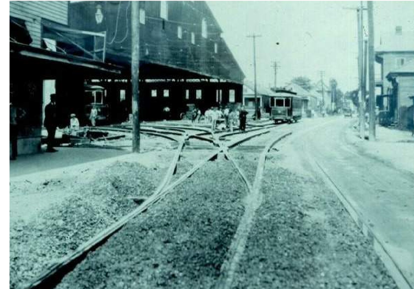
4 ARBELLA STATION TRACKS 1920s N.T.S.
