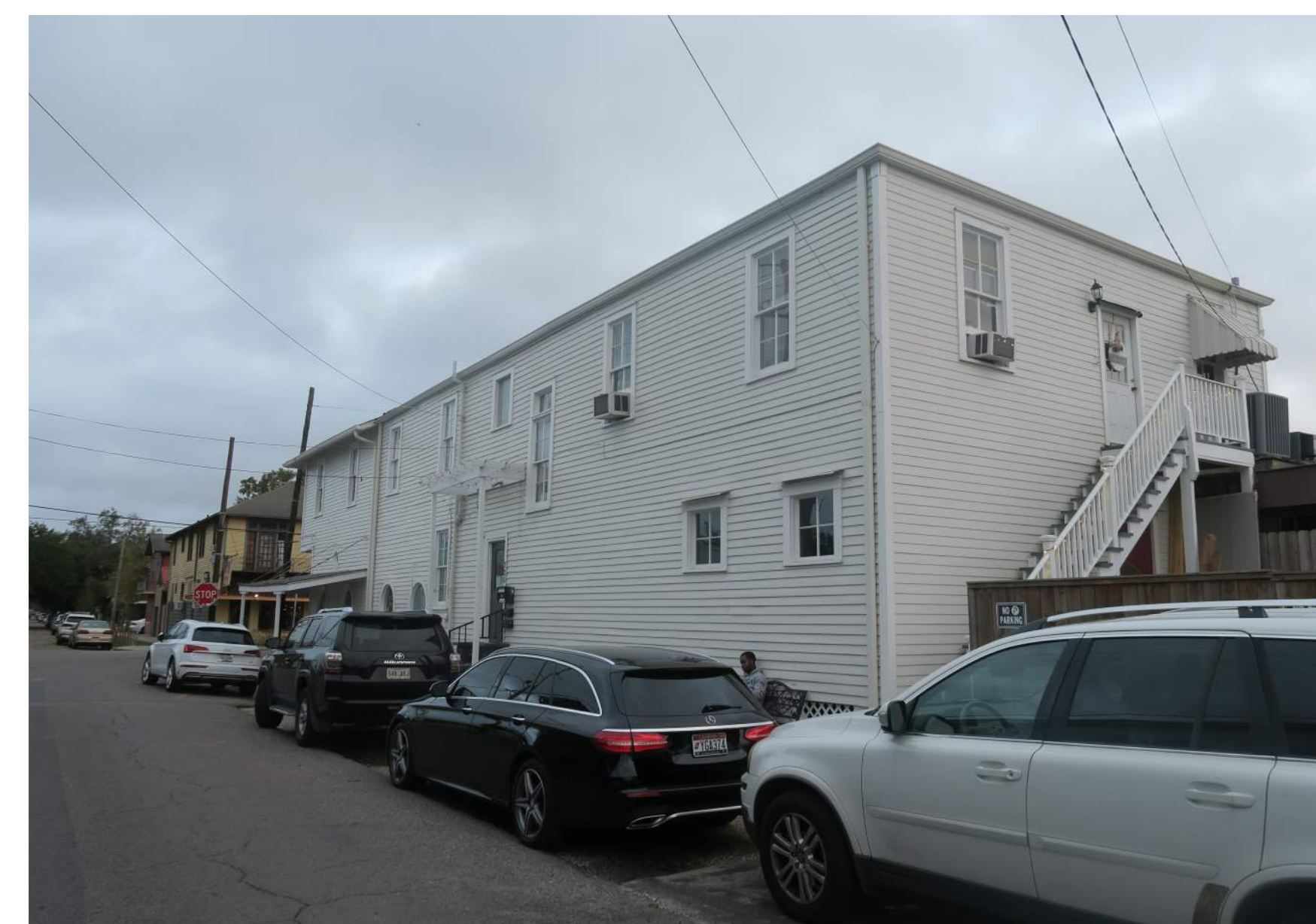
8 EXISTING CONDITIONS BACK VIEW FROM JOSEPH STREET N.T.S.
