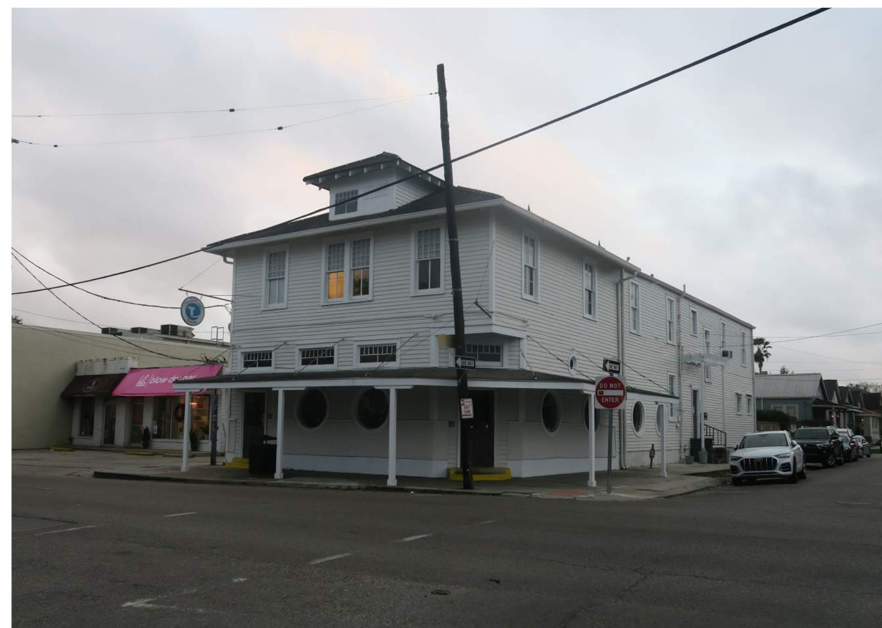
5 EXISTING CONDITIONS FRONT VIEW FROM MAGAZINE STREET N.T.S.
