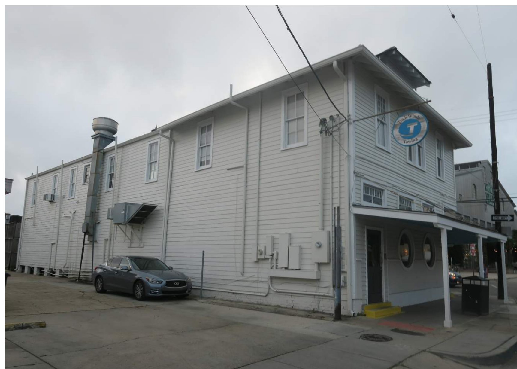
7 EXISTING CONDITIONS SIDE VIEW FROM SIDE PARKING LOT N.T.S.
