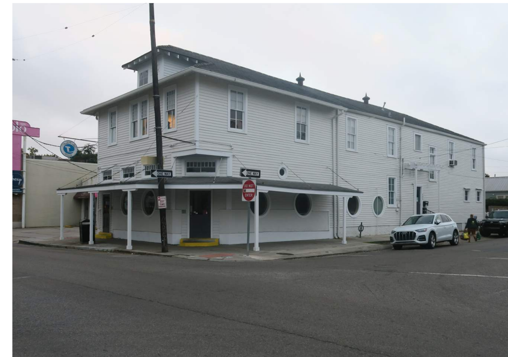
6 EXISTING CONDITIONS SIDE VIEW FROM JOSEPH STREET N.T.S.
