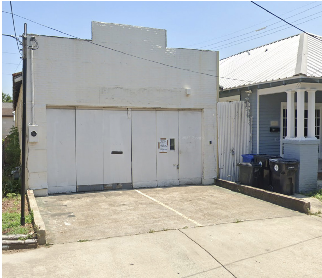
Existing Building Photo Oak Street
