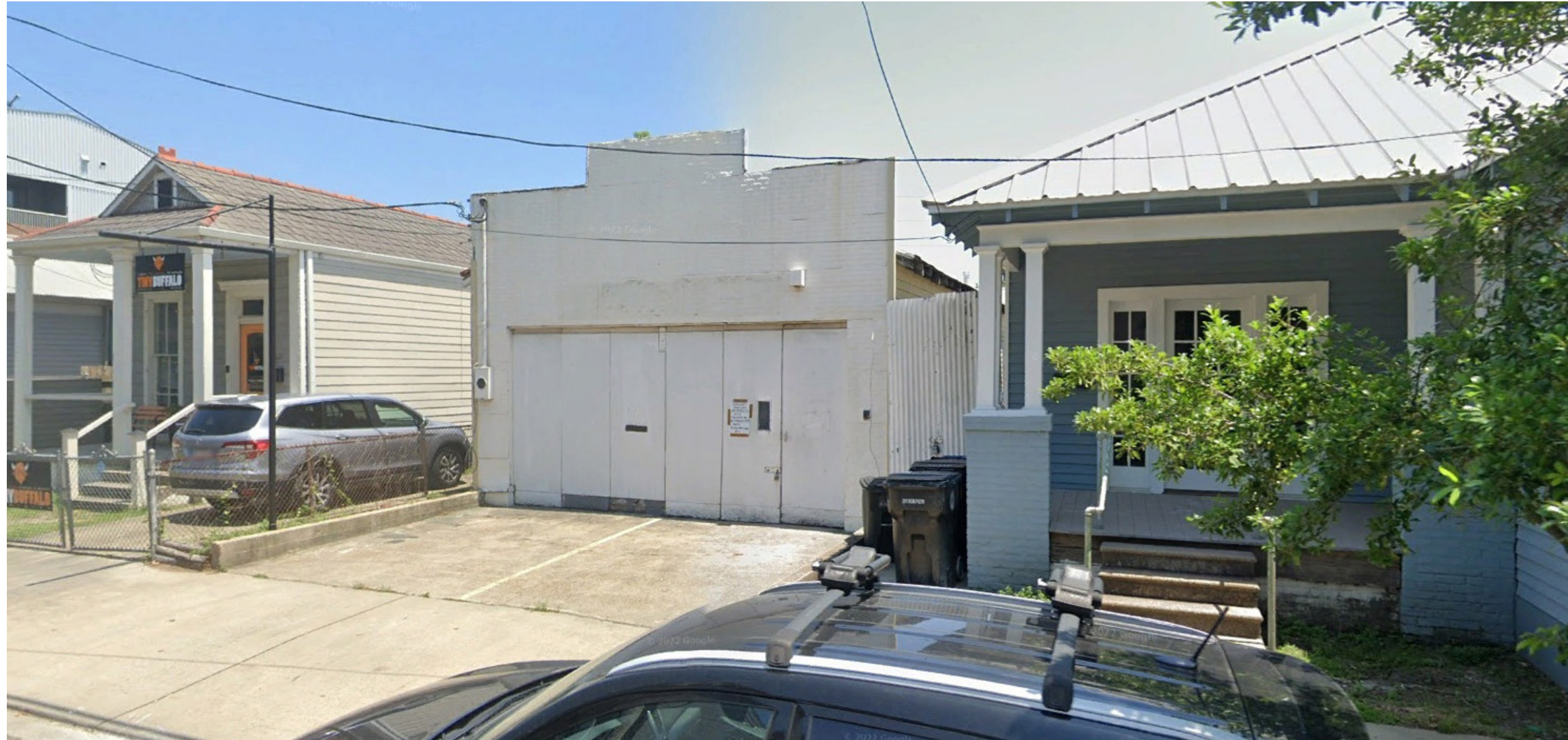
Existing Building Photo Oak Street
