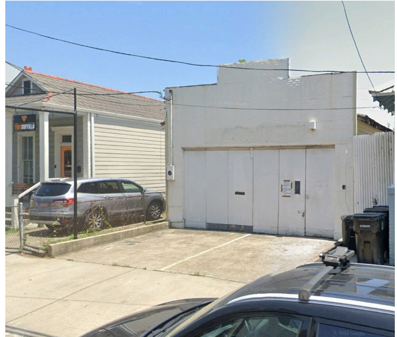
Existing Building Photo Oak Street
