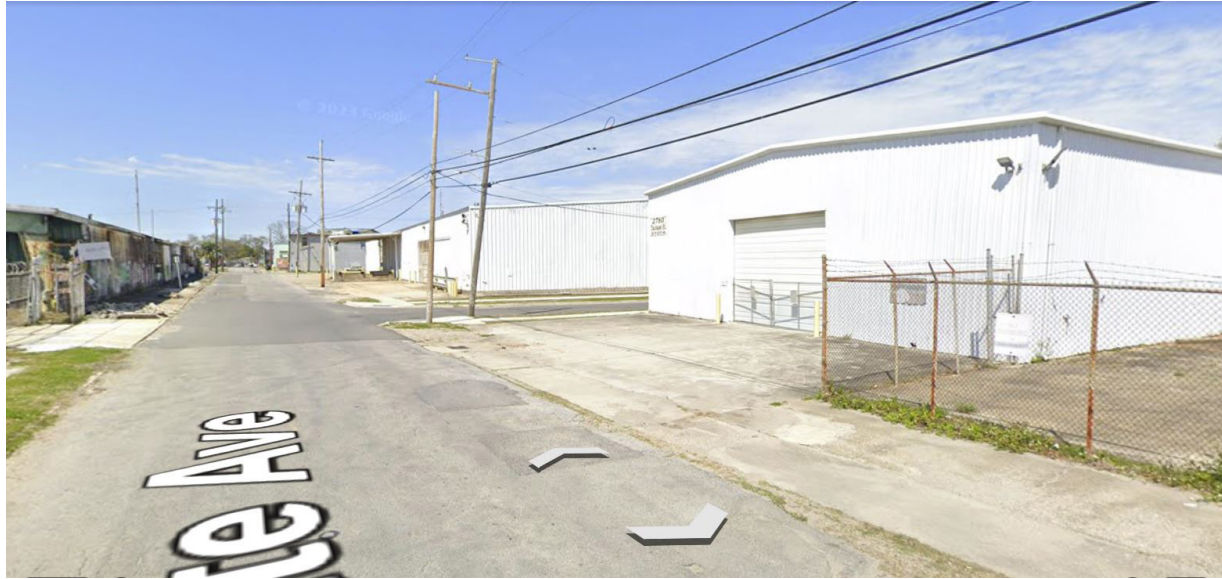
View facing north-west of existing industrial warehouses along Lafitte Ave.
