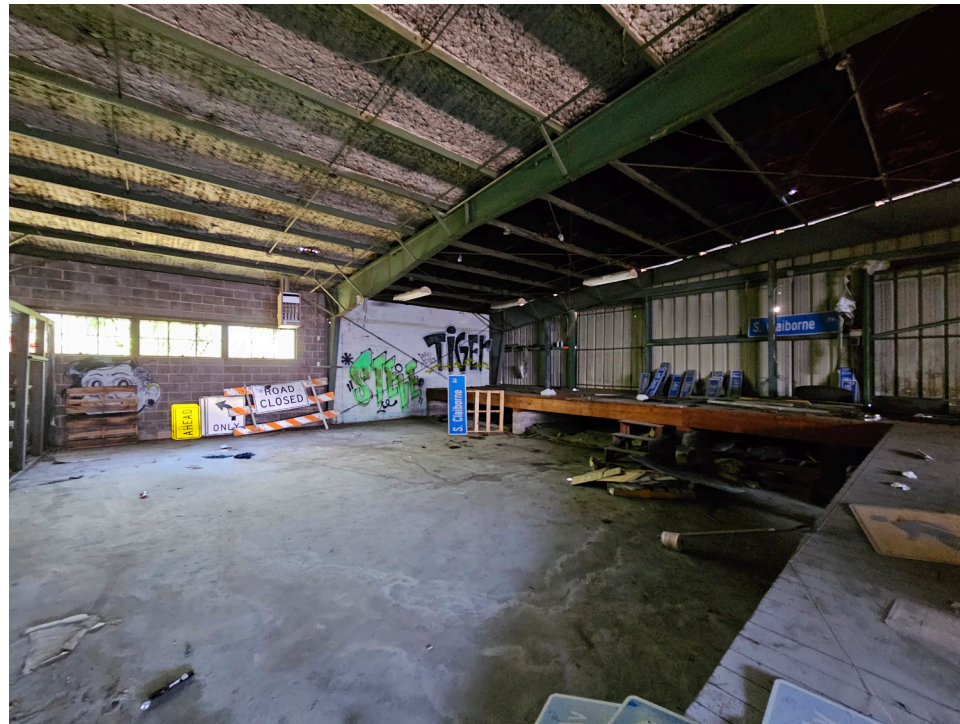
Existing warehouse building interior view looking east.
