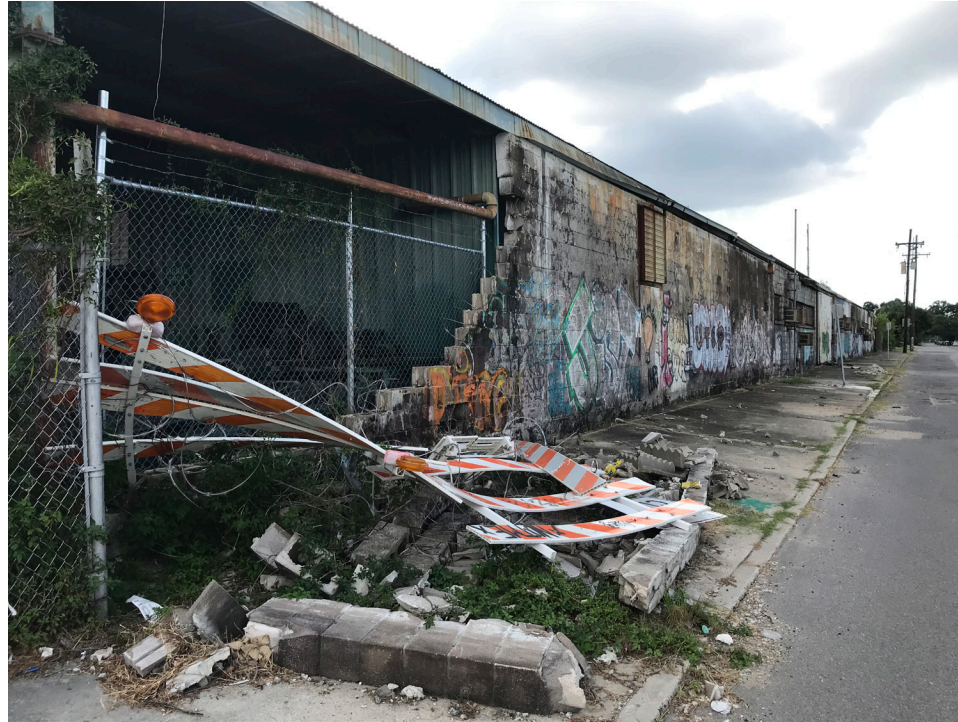
Existing warehouse building facade looking north-west along Lafitte Ave.
