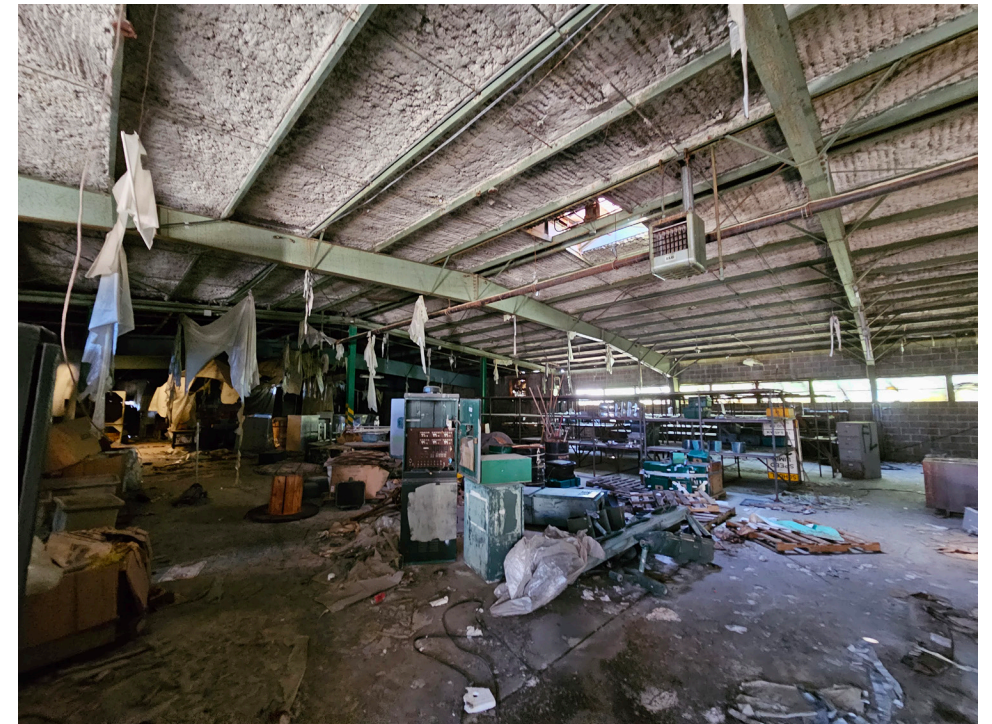
Existing warehouse building interior view looking south.
