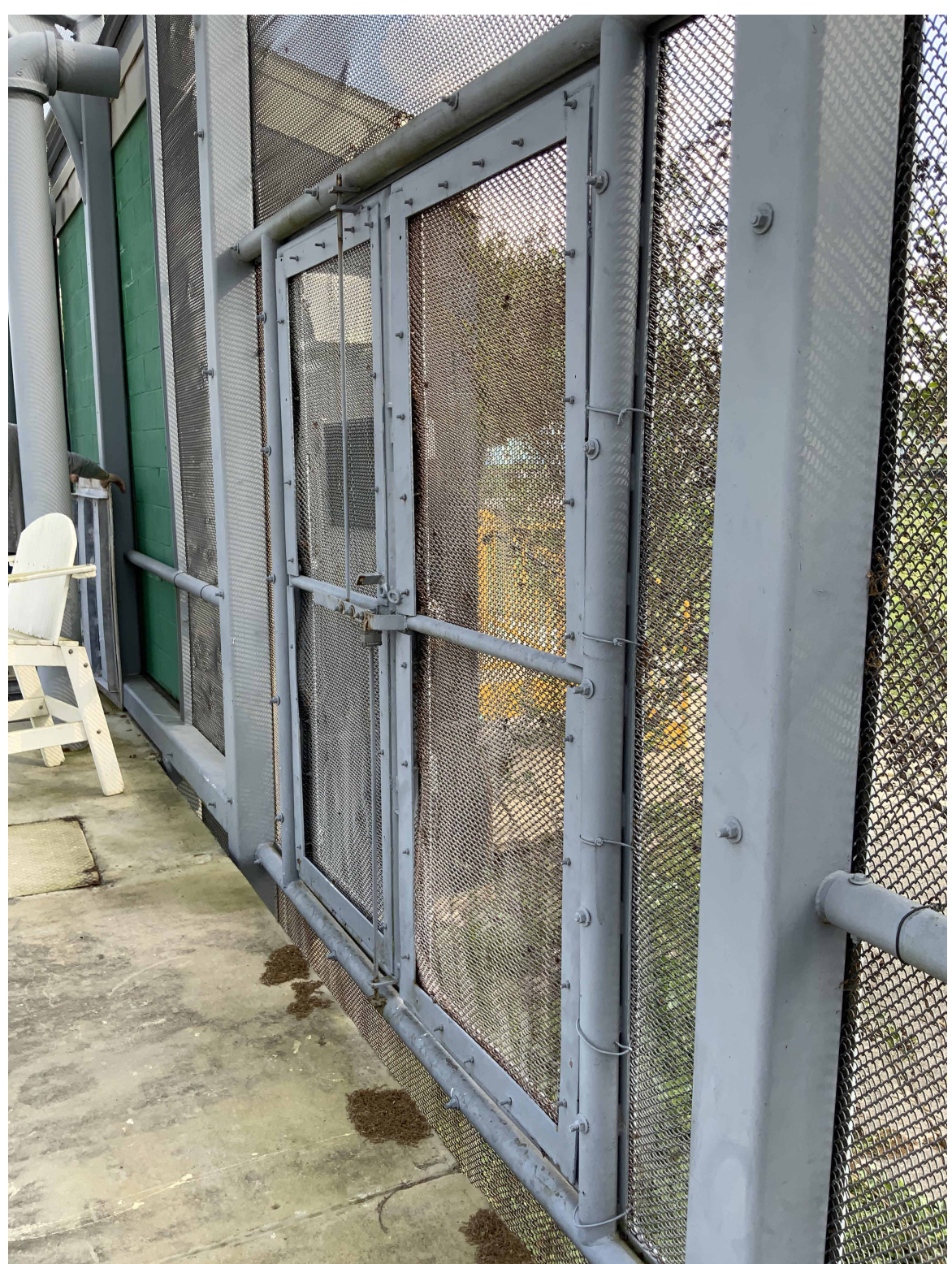
EXISTING PHOTO 7 12" = 1'-0" B3
