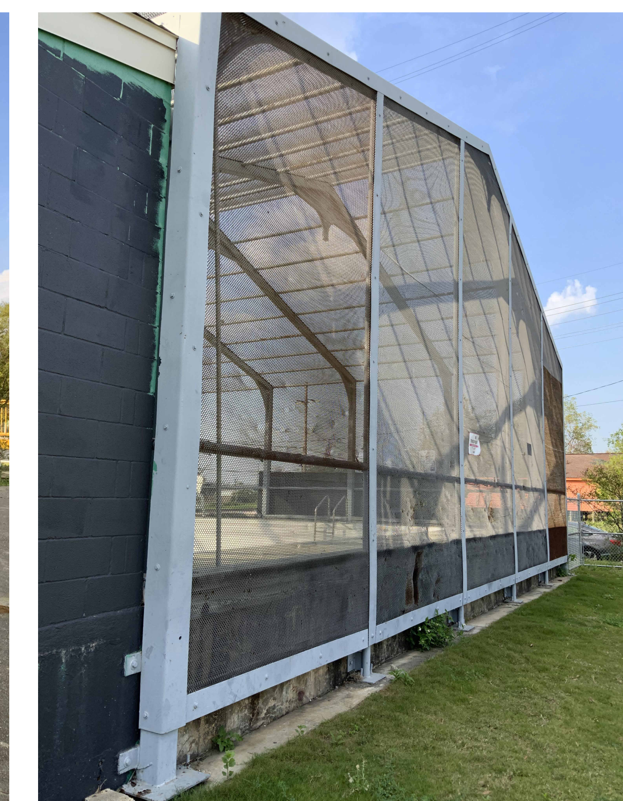
EXISTING PHOTO 5 12" = 1'-0" B1
