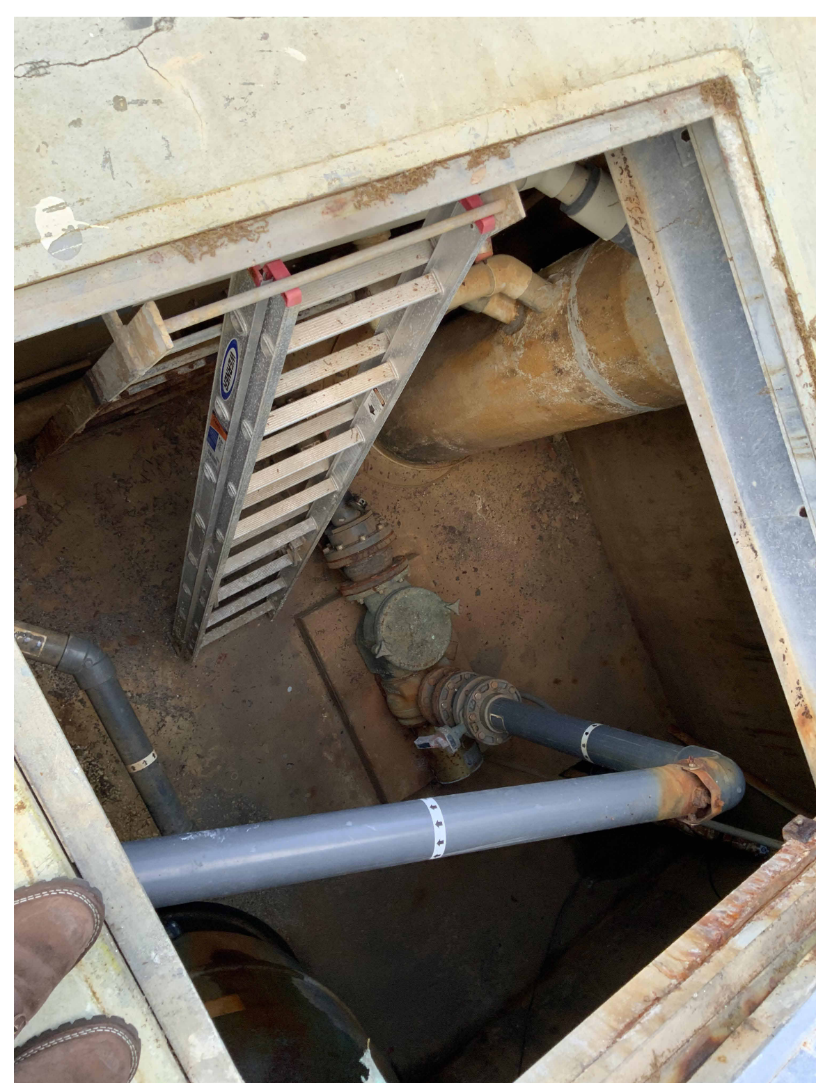
EXISTING PHOTO 8 12" = 1'-0" B4
