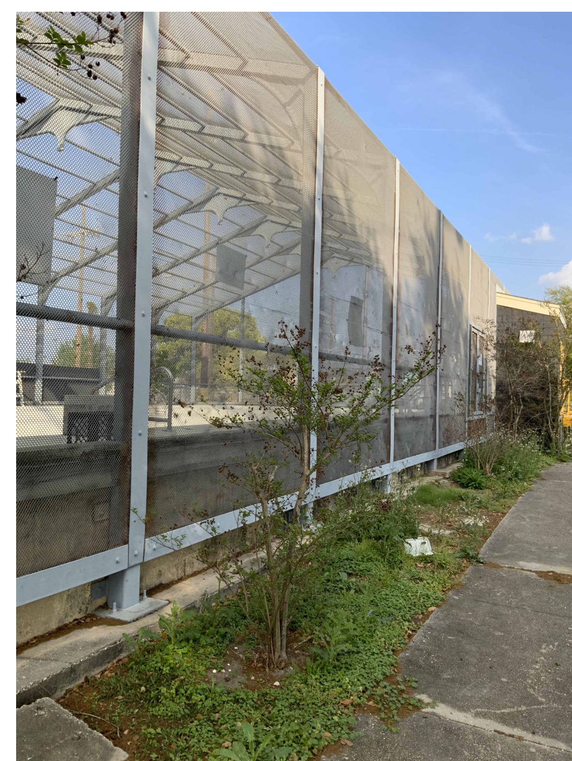
EXISTING PHOTO 6 12" = 1'-0" B2
