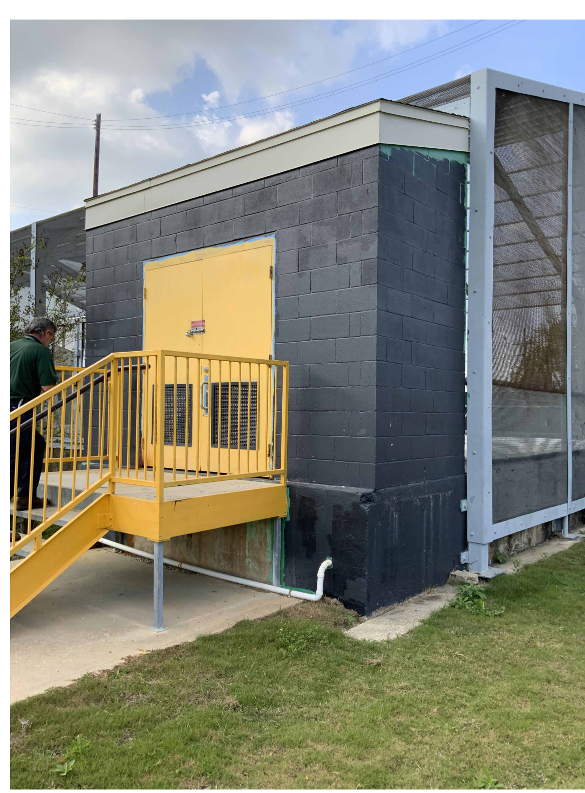
EXISTING PHOTO 2 12" = 1'-0" A2
