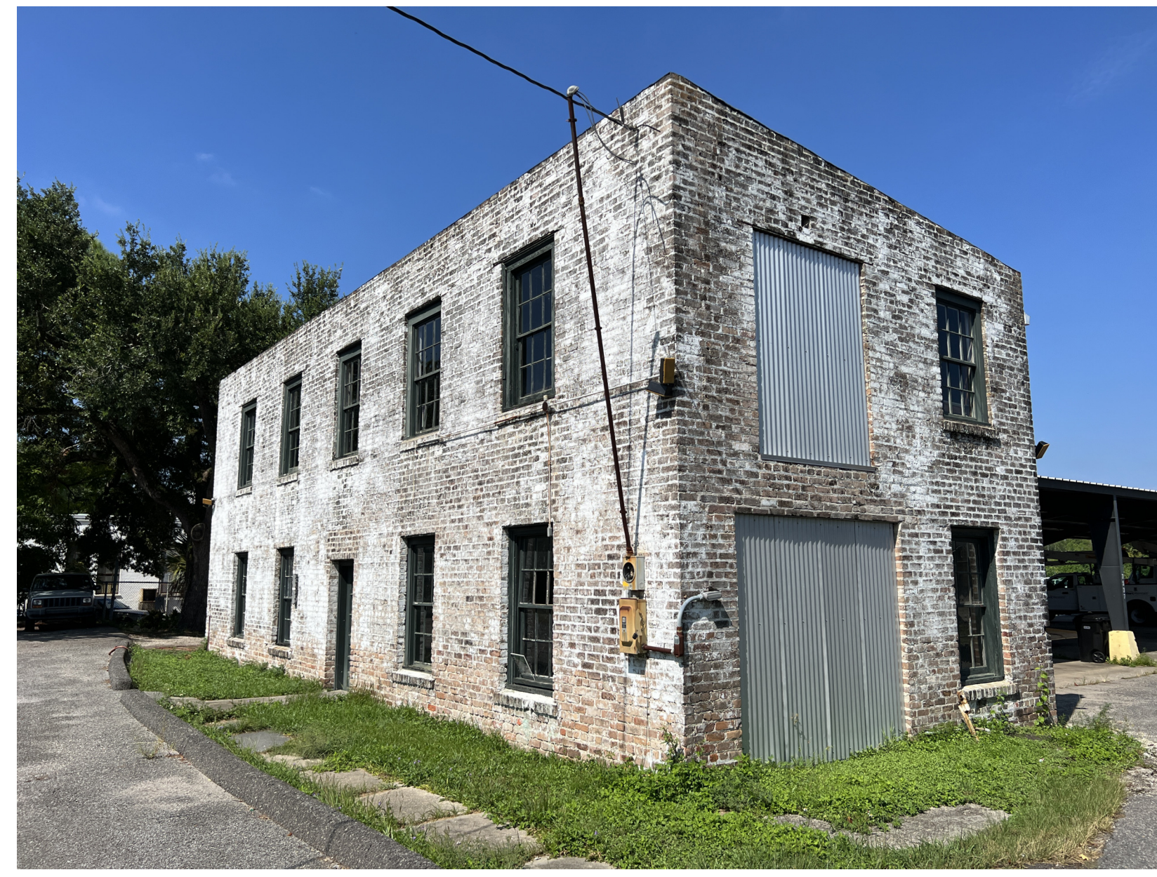
SOUTH AND EAST ELEVATIONS
