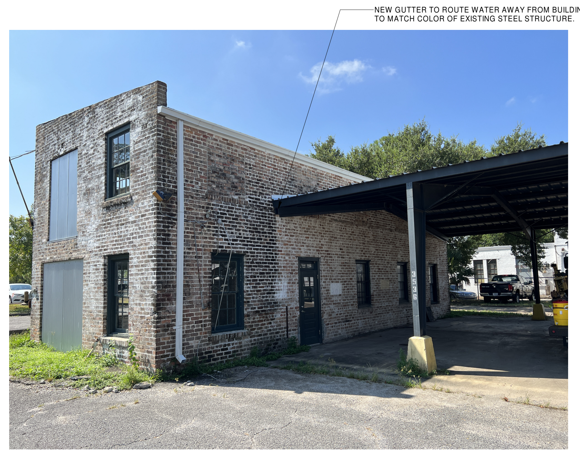
NEW GUTTER LOCATION
