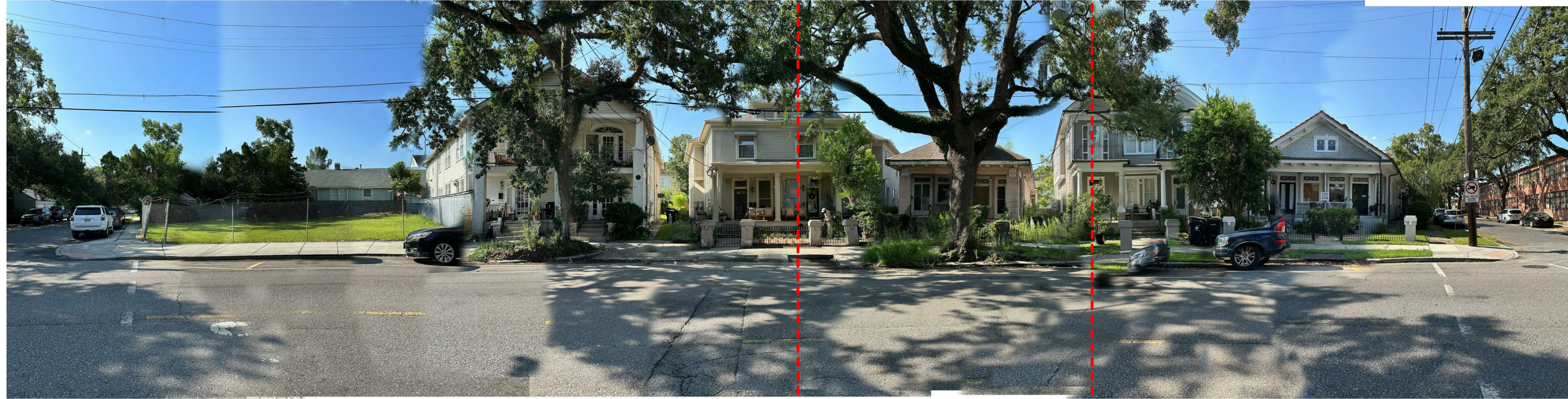
TOWARD DOWNTOWN ACROSS STREET LOCATION TOWARD UPTOWN MAGAZINE STREET
