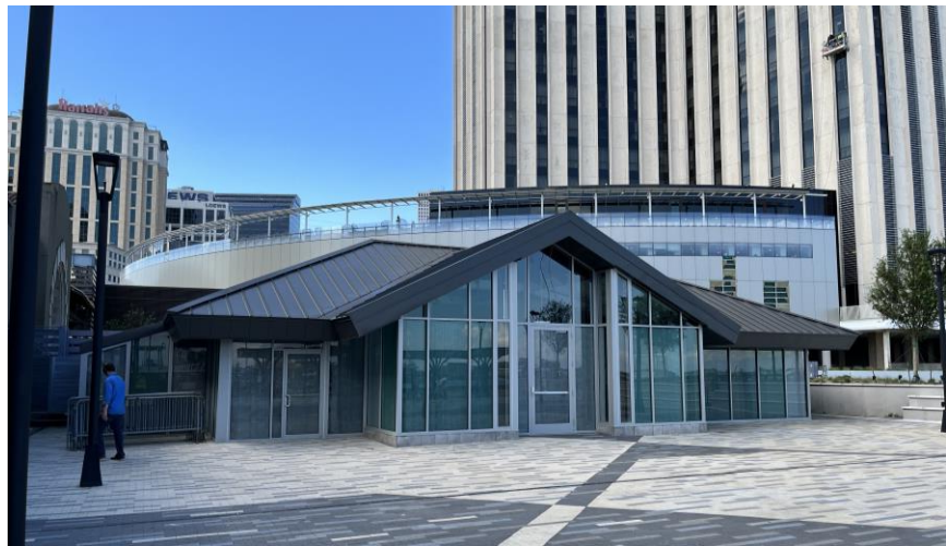
Existing Restaurant view
