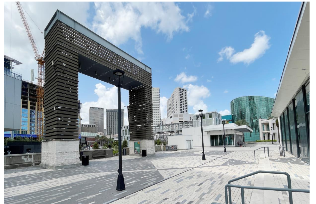
Existing Canal Street Portal view
