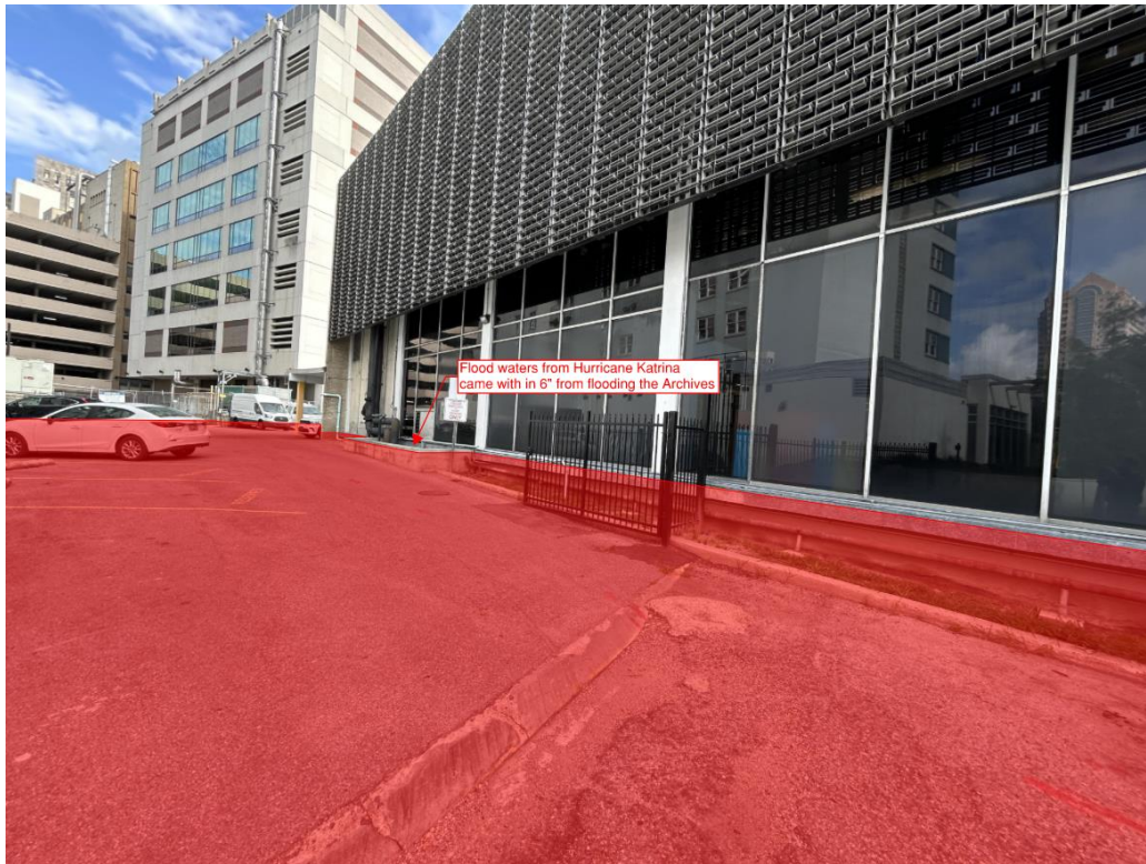
Exterior Water Line
