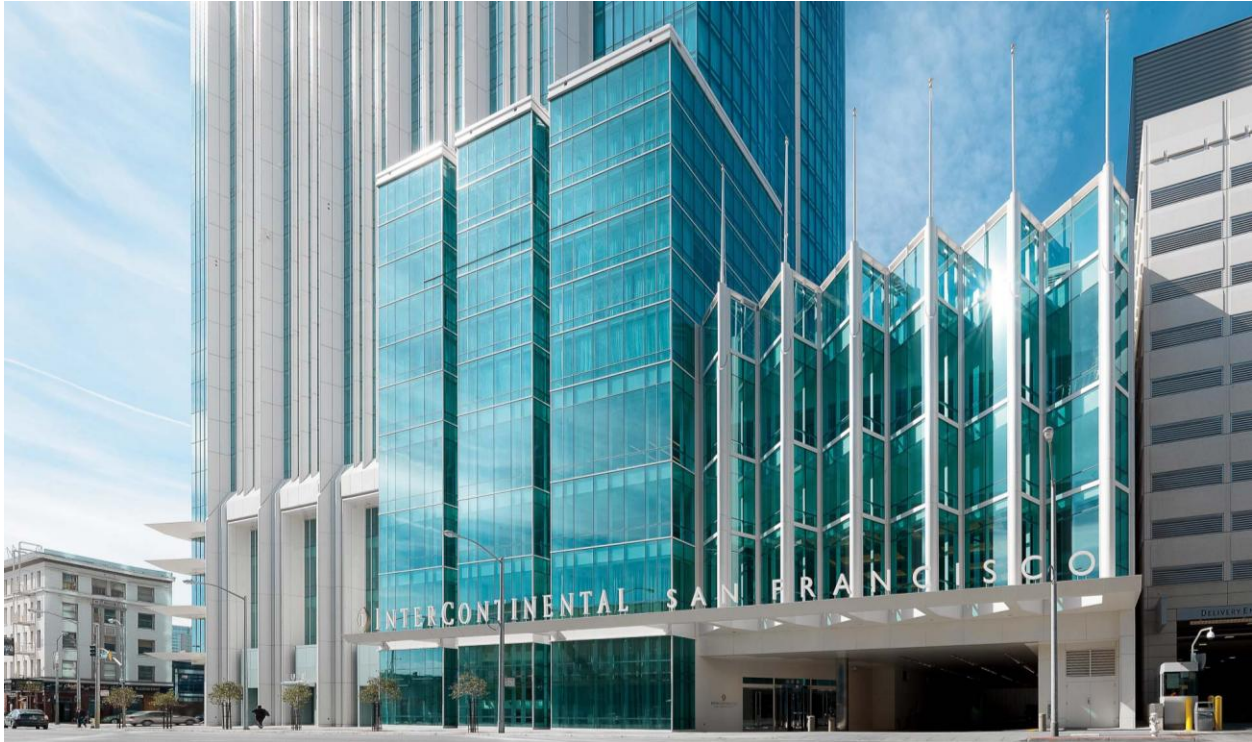
Figure 13. A portion of TDRs from The Old Mint were used to develop the InterContinental San Francisco Hotel. Image courtesy of Continental Development.
