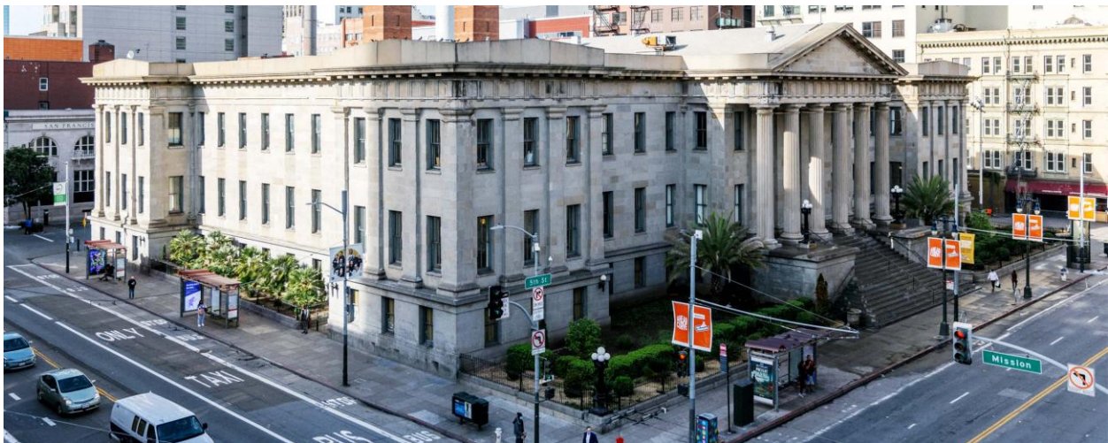
Figure 12. The Old Mint, a venue in San Francisco completed as a branch of the United States Mint in 1874, was renovated through profit from TDR in the early 2000s. Photo courtesy of Non Plus Ultra.
