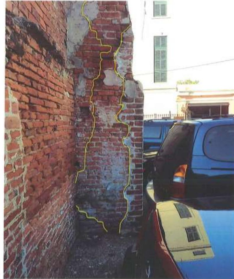
Photo #6-View of cracked section of southwest wall
