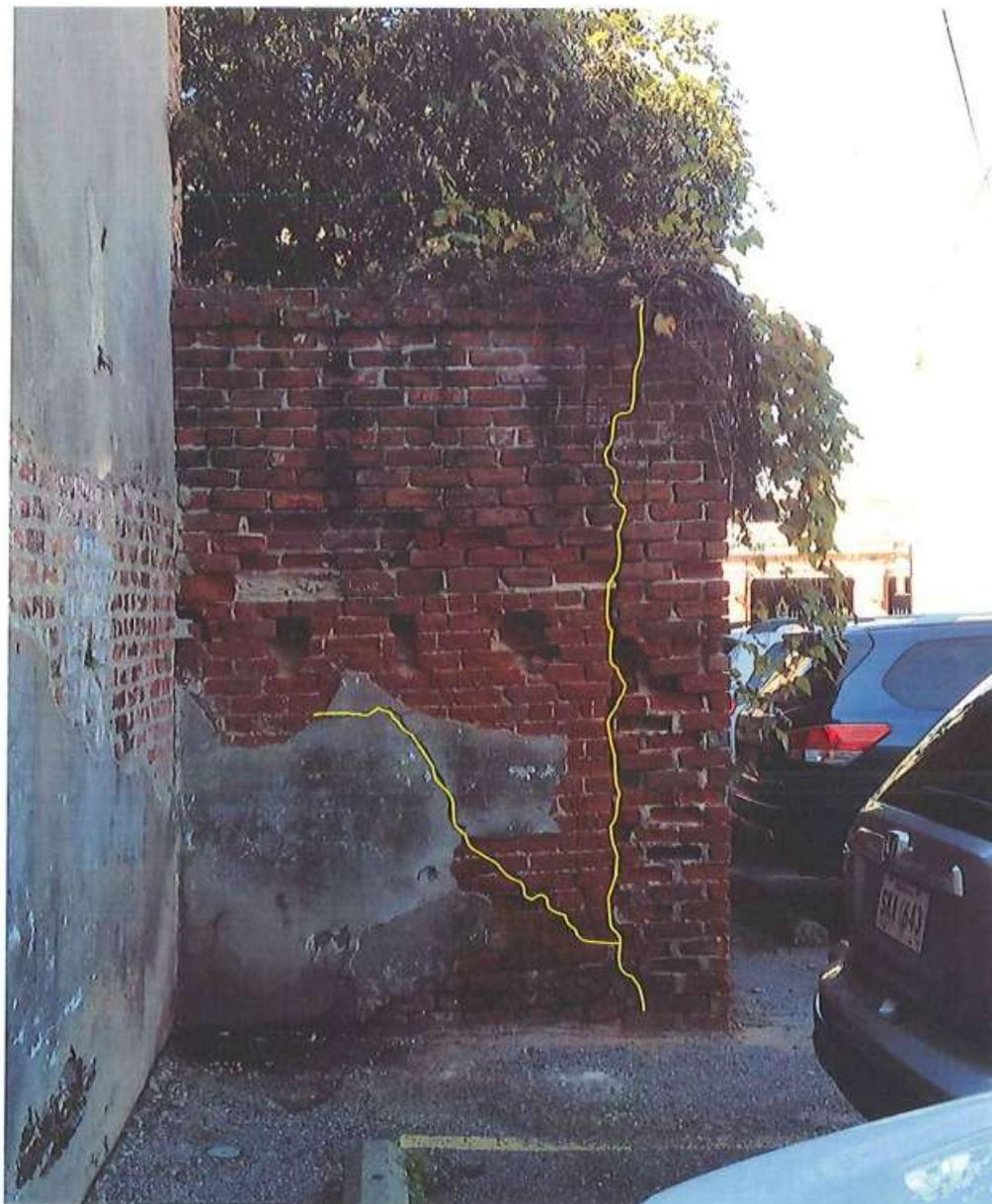
Photo #5-View of cracked section of southwest wall
