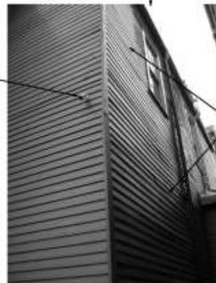
THRU-WALL EXHAUST VENT FOR RESTROOM TO BE LOCATED @ THIRD FLOOR
