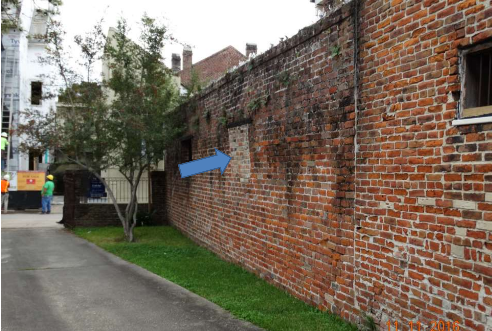
905 Governor Nicholls – In-filled window opening
