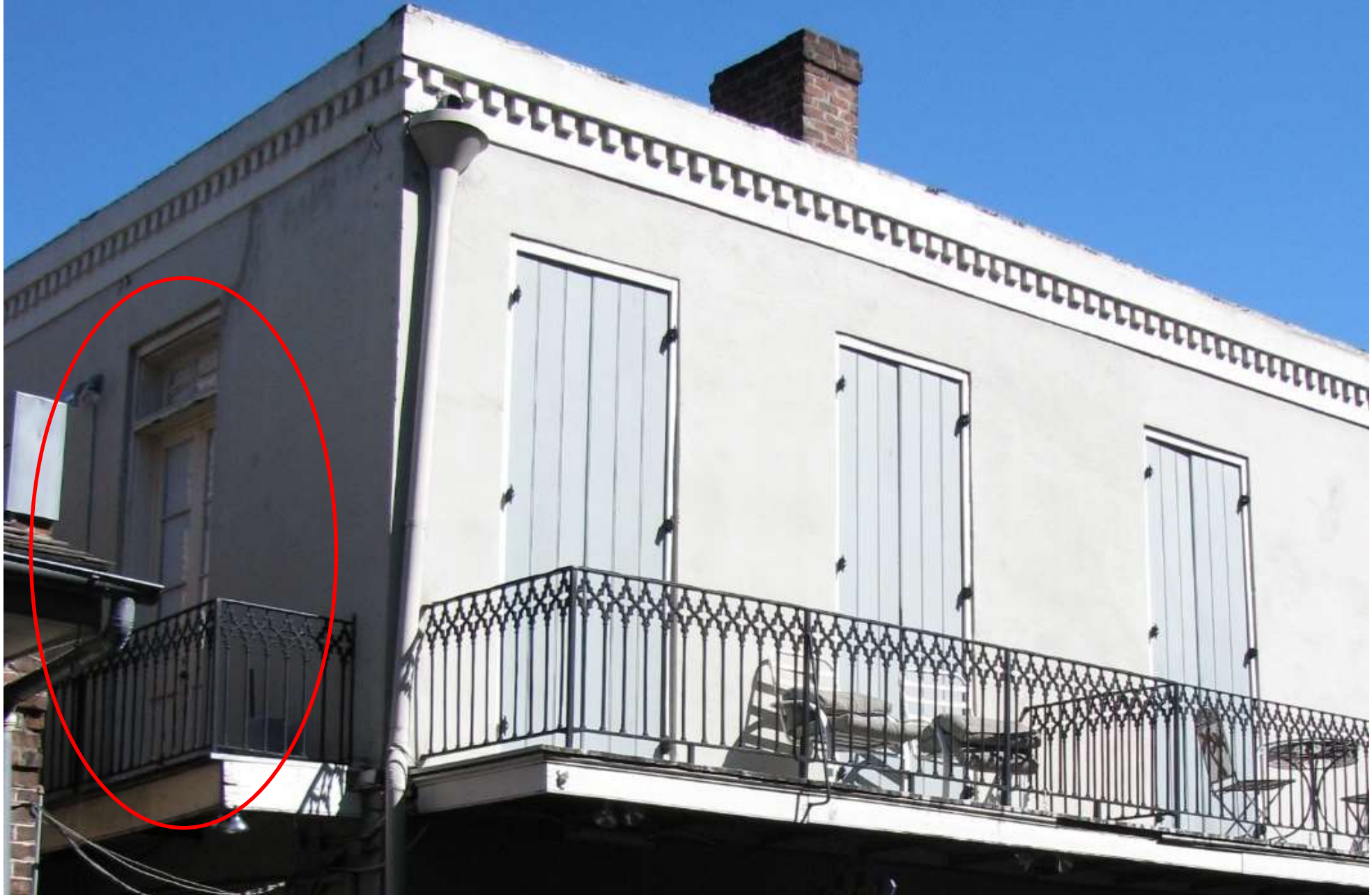
811 Toulouse – 2009 Prior to Awning Installation
