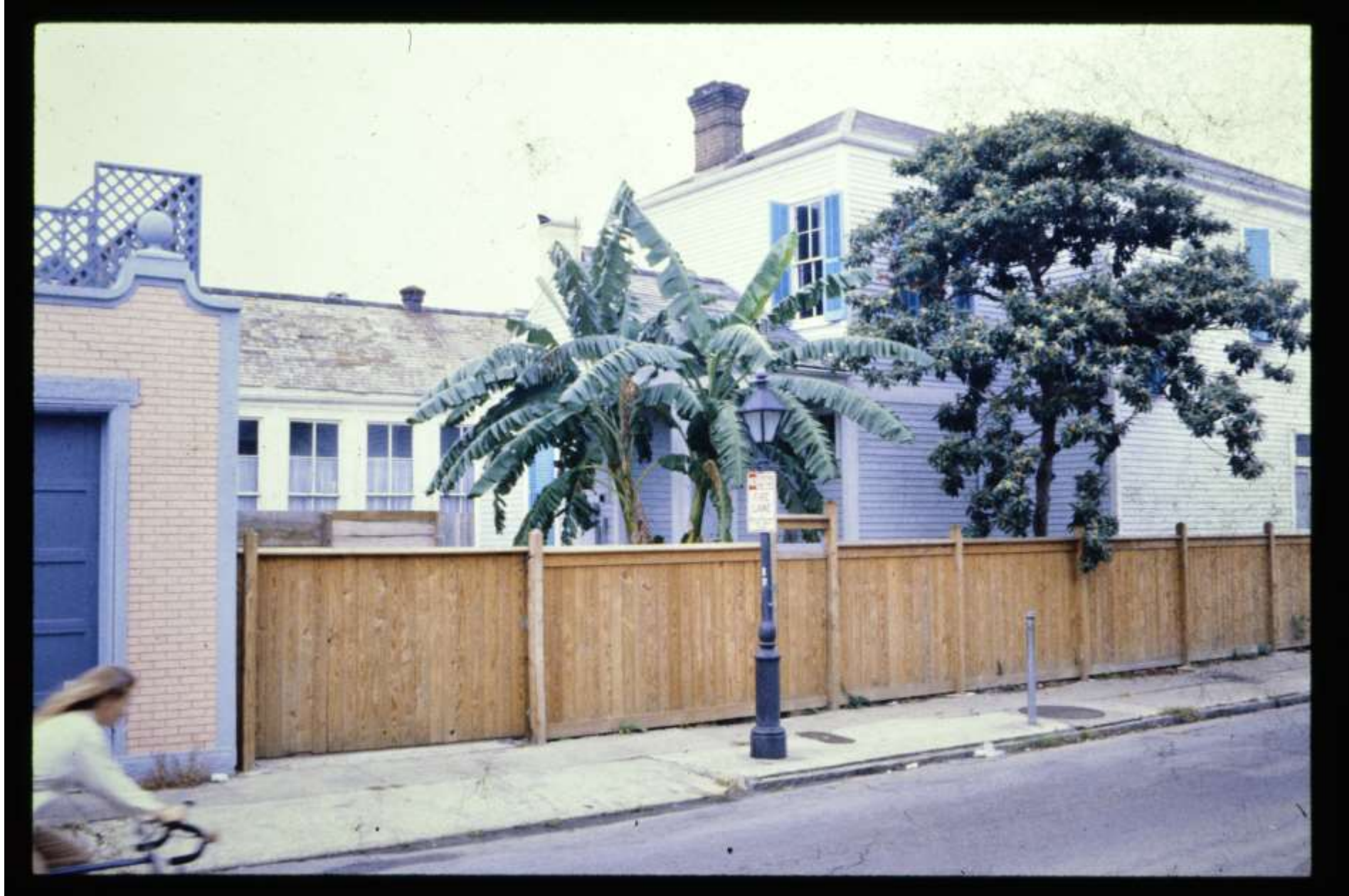
1240 Royal – 1986 – Prior to rear addition
