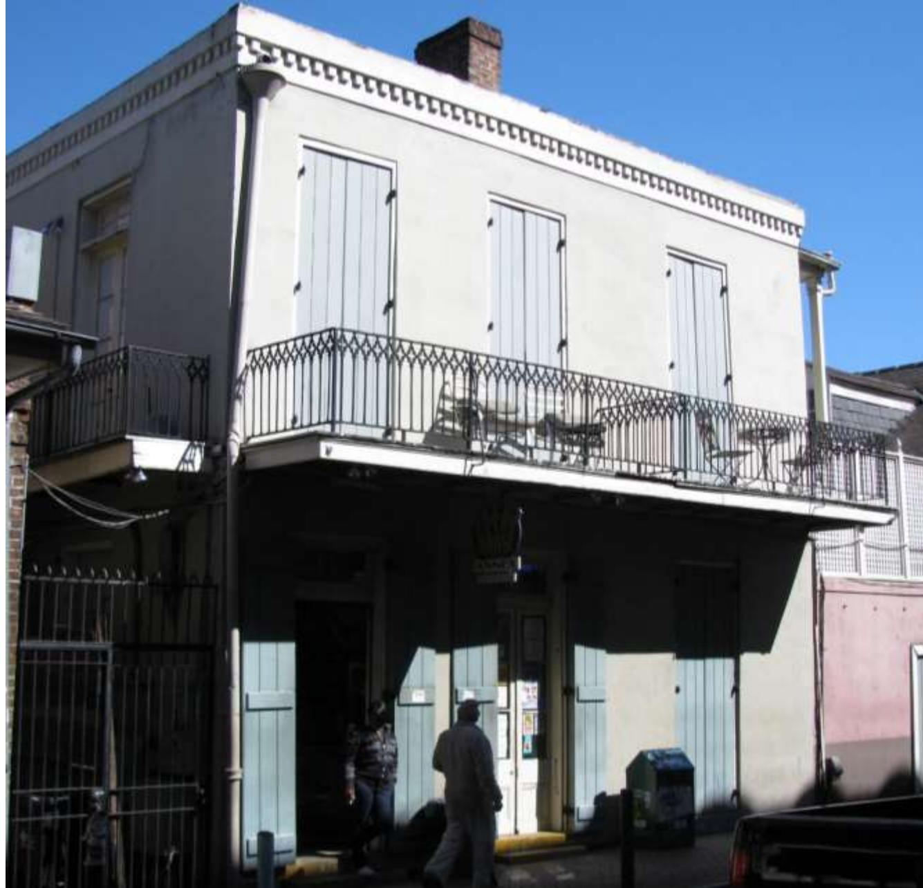
811 Toulouse – 2009 Prior to Awning Installation
