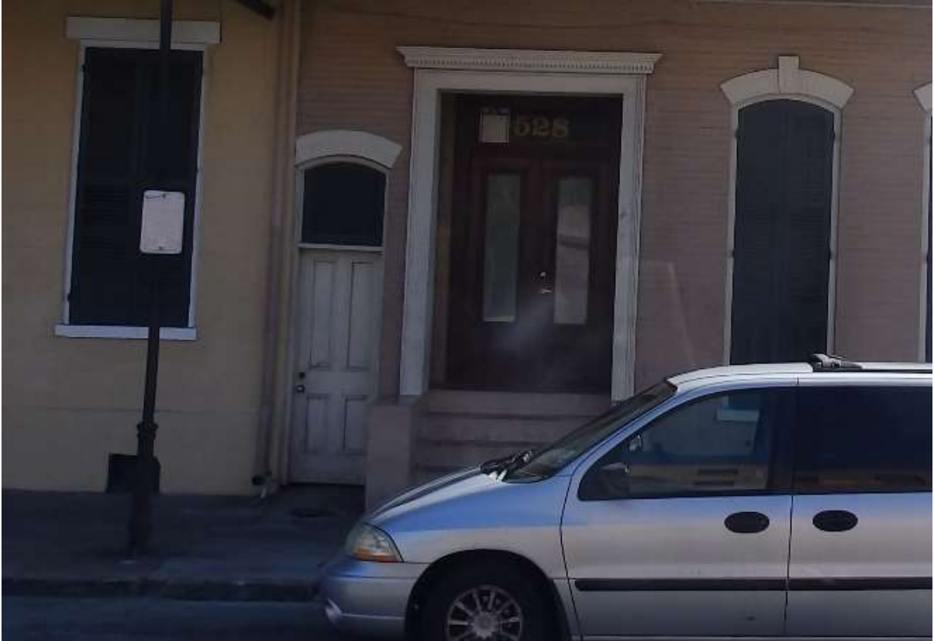
528 N Rampart – Alleyway door in 2014
