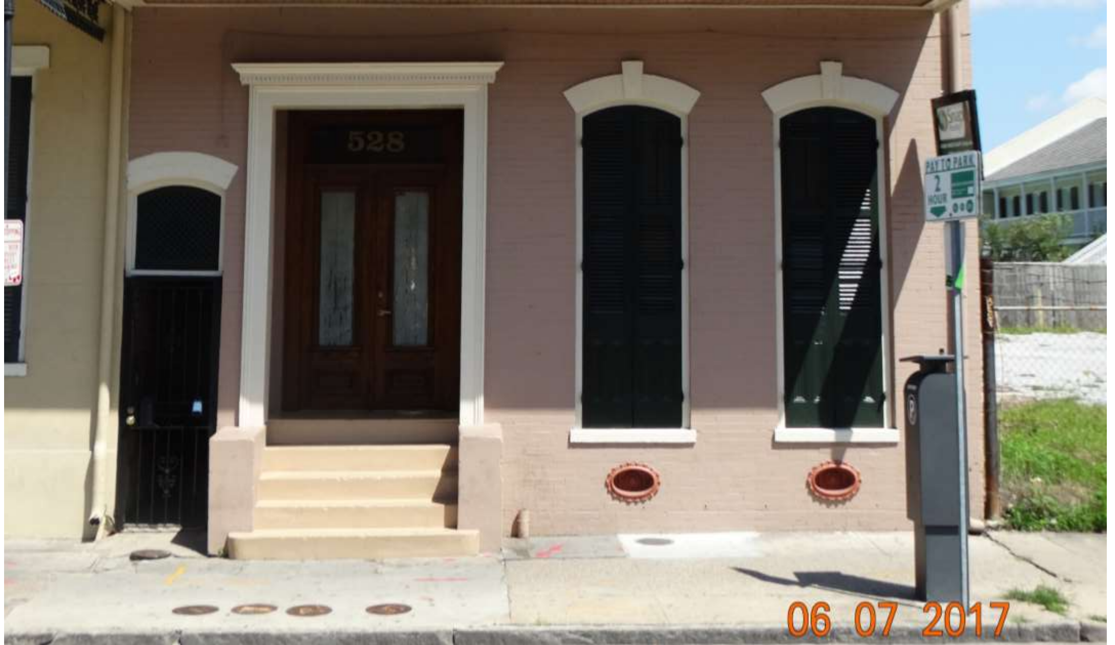
528 N Rampart – Alleyway gate installed without permits
