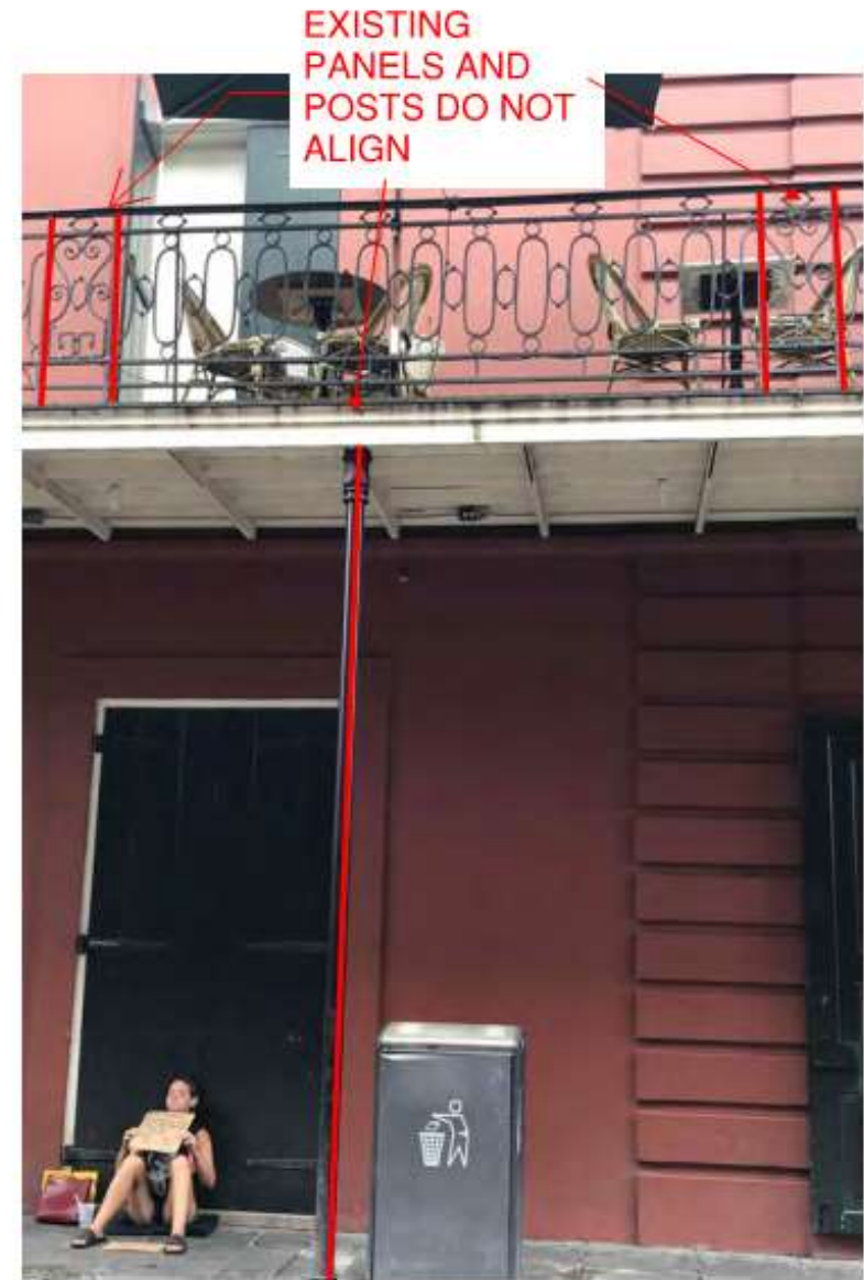
EXISTING IRON RAILING COLUMN CONDITION ST. PETER SIDE
