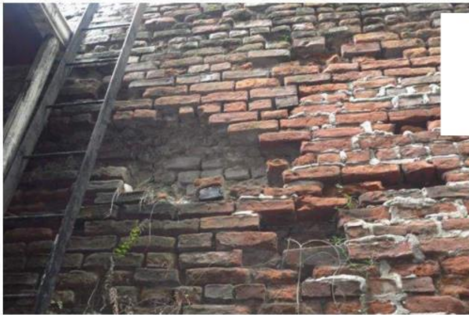
Enlarged photo shows the observed condition of the two non-bonded walls.
