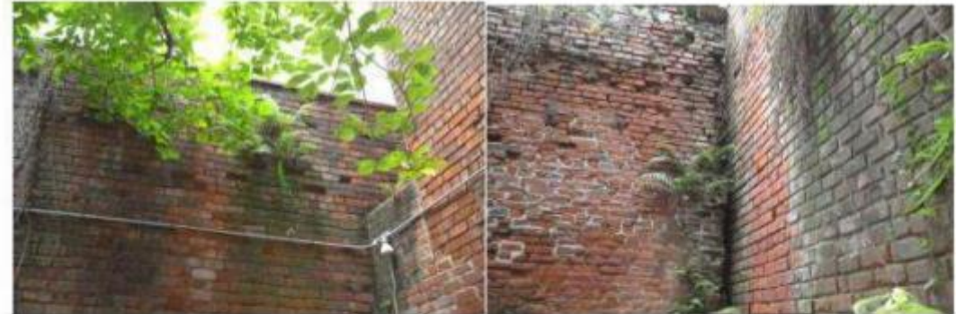
More cracks at the wall and the wall connection
