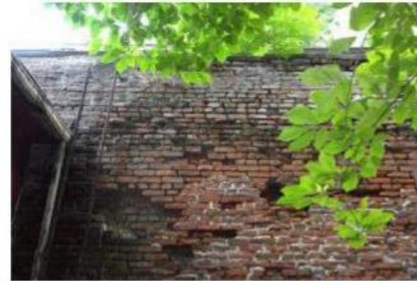
left side wall detail of the missing bricks
