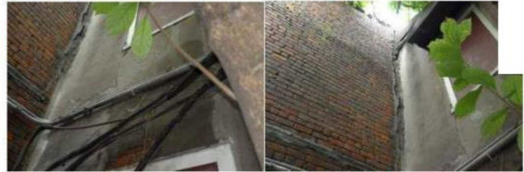
Continuous cracks at the gable wall of the rear two story building
