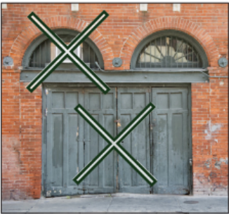
Doors and/or openings should not be modified to install a new non-historic door type. In this case, two door openings were combined and jambs infilled for the installation of the large central door.
