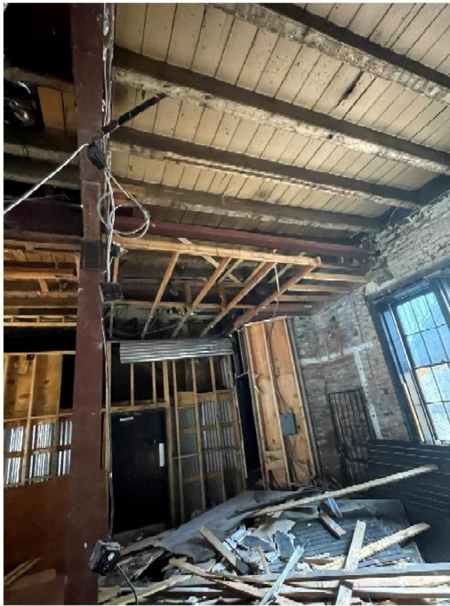
Picture 8. Existing double angle tieback to remain. Tuckpointing repair necessary at exterior masonry.
