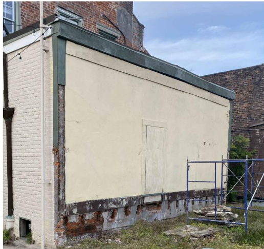
③ PHOTOGRAPH OF EXISTING STUCCO FINISH ON EXTERIOR MANSION WALL
