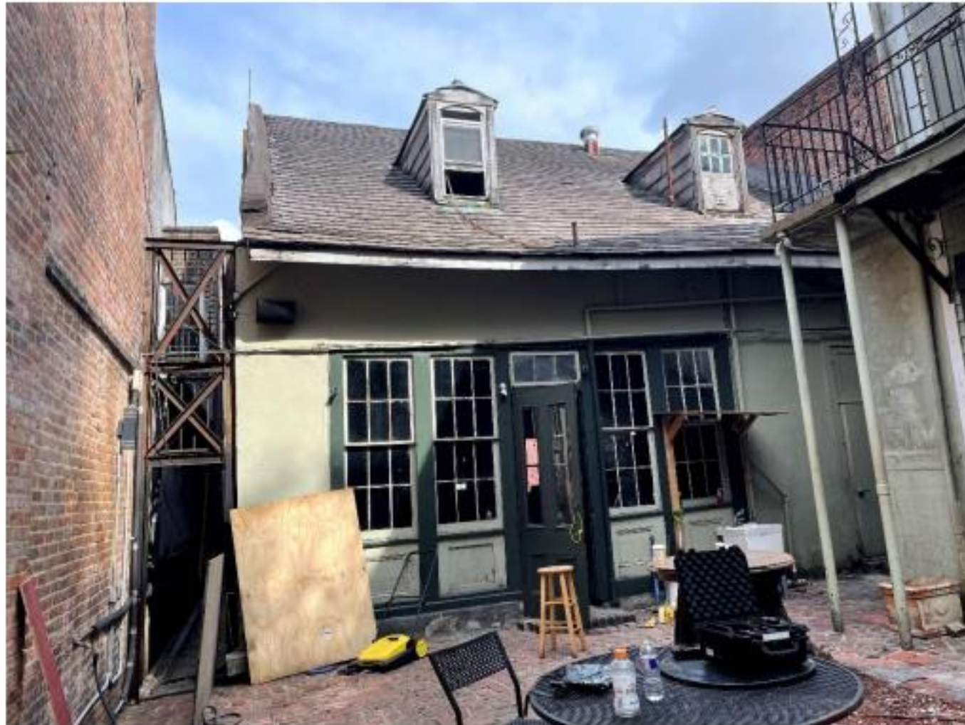
Picture 6: Rear opening of building to have channel lintel installed (taken from exterior)
