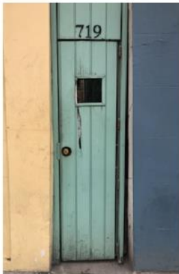
5 DETERIORED SHUTTERS/ DOORS
