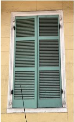
5 DETERIORED SHUTTERS
