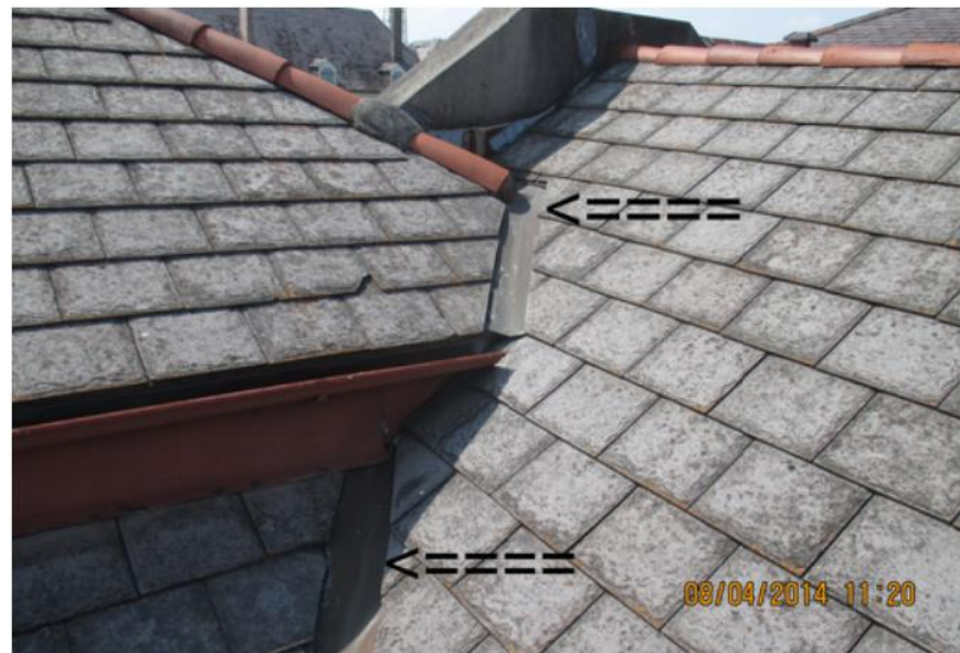
Replace firefree with new slate roof from this valley around the courtyard.
