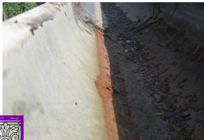
Rusted out galvanized gutters to be replaced with copper gutters.
