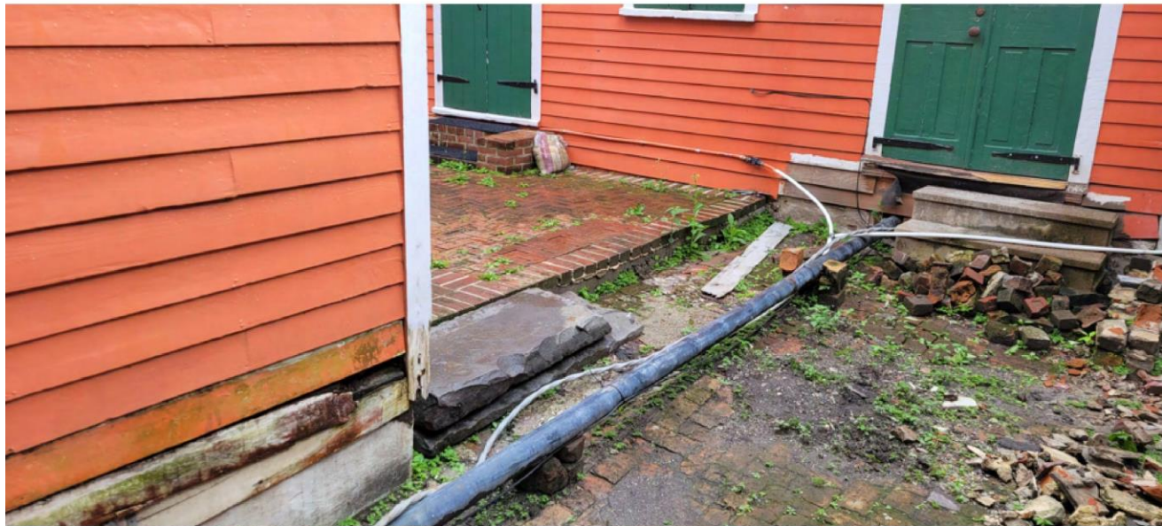
1116 Rear middle courtyard has mis-matched elevation with exposed sewage and water lines
