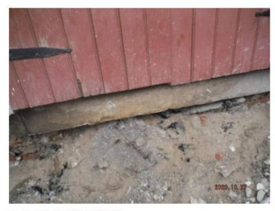
Photo 3: DAMAGED/MISSING FOOTING
