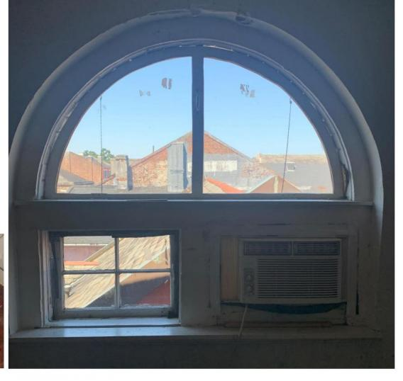
Third floor arched window to be restored and reinstalled in window. Window unit to be removed and four light window to be reinstalled.
