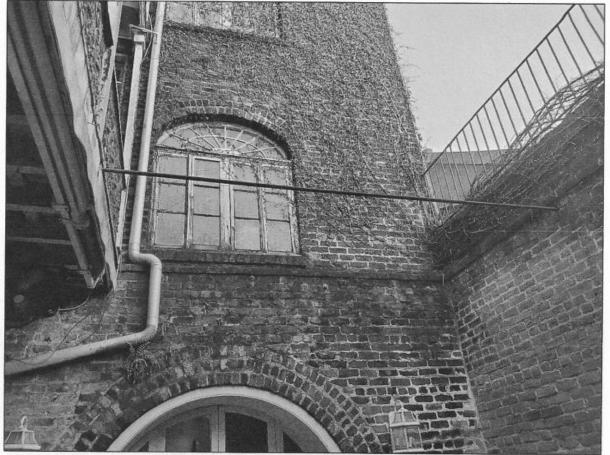
Picture of existing tie rod between masonry wall and 2<sup>nd</sup> floor balcony – Looking towards building
