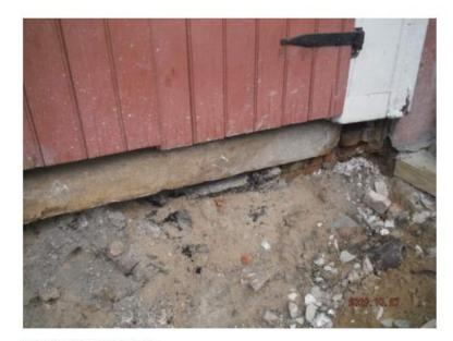
Photo 4: DAMAGED FOOTING.
