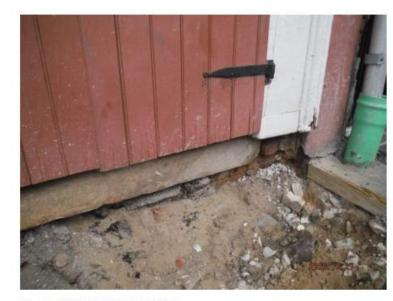
Photo 2: DAMAGED/MISSING FOOTING.
