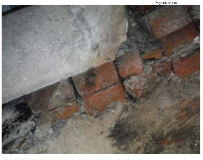
Photo 7: CLOSE UP OF DAMAGED AND DISPLACED BRCIK IN FOOTING.
