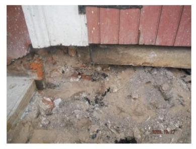
Photo 1: DAMAGED FOOTING
