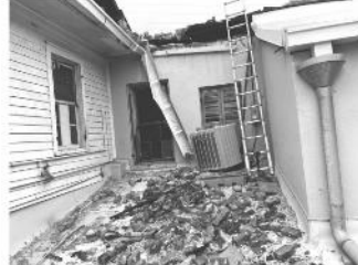
AERIAL VIEW OF BRICKWORK ON EXISTING ROOF STRUCTURES AND DAMAGED GUTTER
