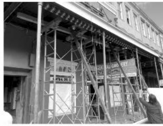
STREET FRONT FACADE WITH TEMPORARY SHORING IN PLACE
