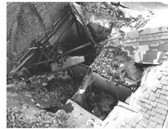
AERIAL VIEW OF COLLAPSED SLATE ROOF
