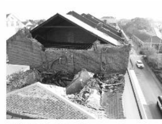
AERIAL VIEW OF COLLAPSED BRICK PARTY WALL
