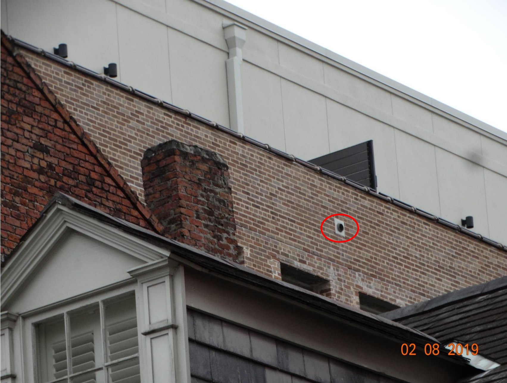
939 Iberville (920 Bienville) – Water Draining onto Neighboring Property
