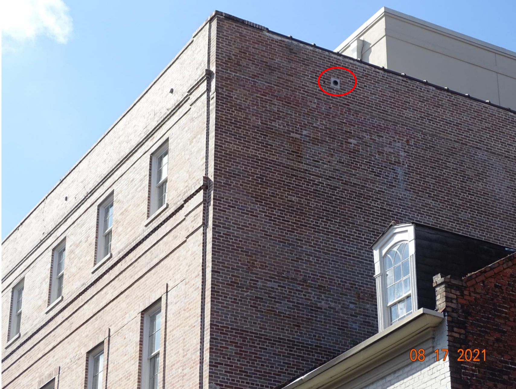
939 Iberville (920 Bienville) – Water Draining onto Neighboring Property
