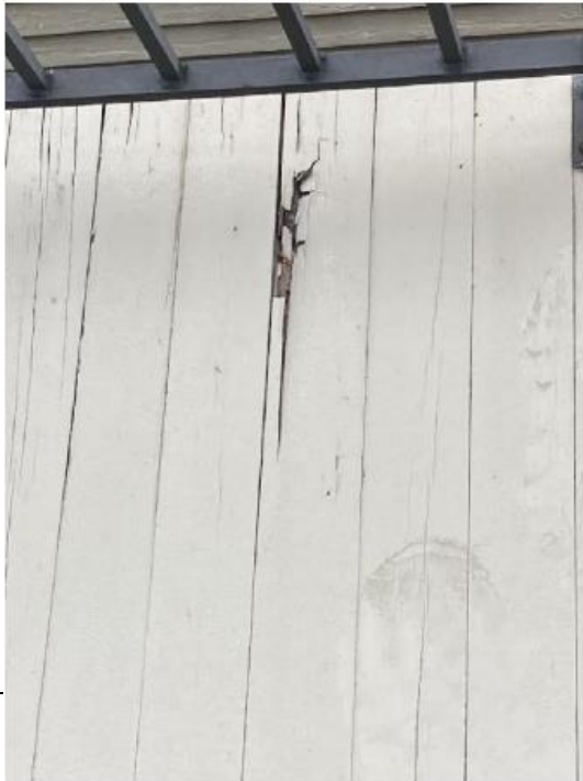
close-up of area showing rotten wood:
