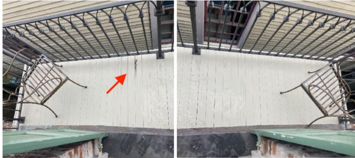
close-up of area showing rotten wood:
