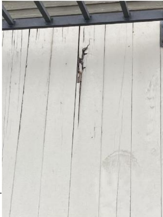
close-up of area showing rotten wood:
