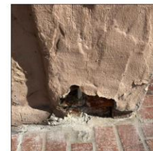
3 Existing Deteriorated Stucco and Bricks
