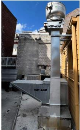
⑤ BLDG 630 - KITCHEN HOOD EXHAUST & SUPPLY FANS
