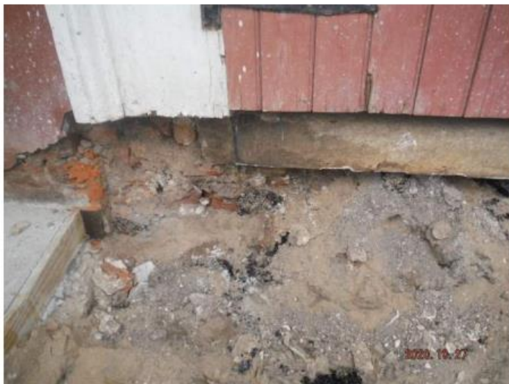
Photo 1: DAMAGED FOOTING
