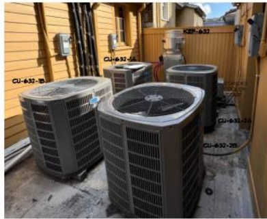
⑦ BLDG 630 (4) A/C COND UNITS, HOOD EXHAUST FAN & COOLER COMP
