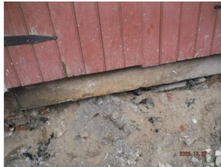
Photo 3: DAMAGED/MISSING FOOTING
