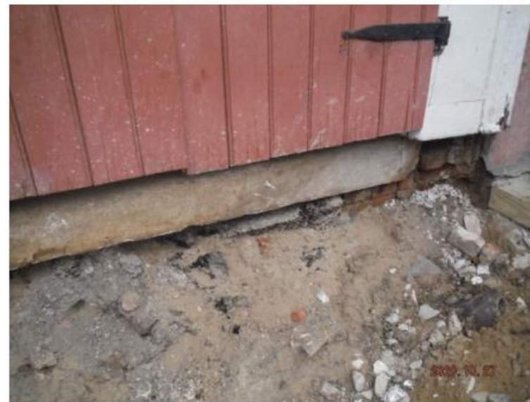
Photo 4: DAMAGED FOOTING.
