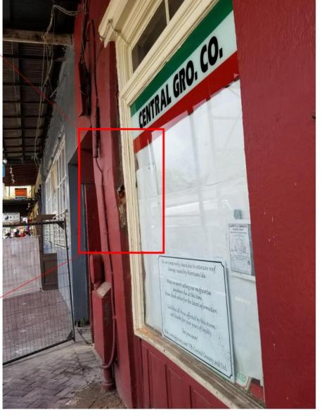
VIEW OF BULGING WALL AT GROUND FLOOR
