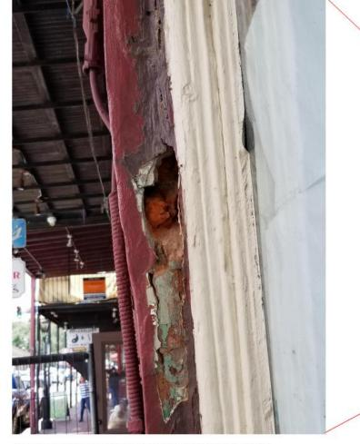
CLOSE UP VIEW OF BULGING WALL AT GROUND FLOOR
