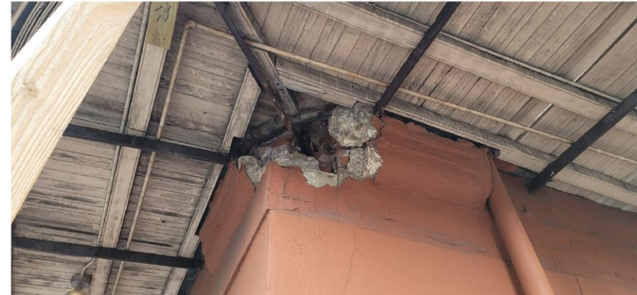
P01 – Image taken from corner of Chartres and Toulouse looking up at damaged balcony, building side; In view is damaged balcony outrigger and multi-wythe masonry wall.
