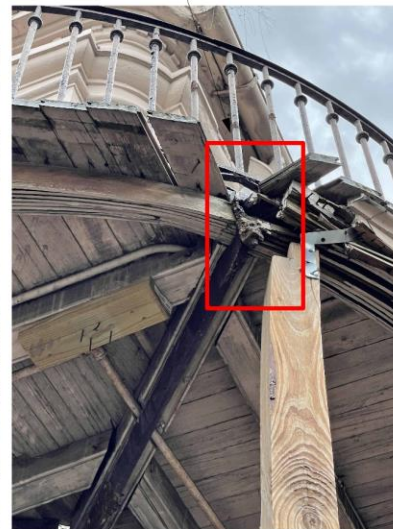
DAMAGED OUTRIGGER
