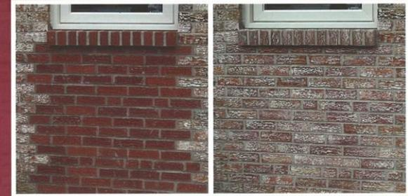
A potassium silicate tint (right) was created to successfully blend the mismatched repair work (left) with the original surrounding brick.
