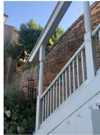
Vegetation on Masonry Walls To Be Removed Scale: NTS
