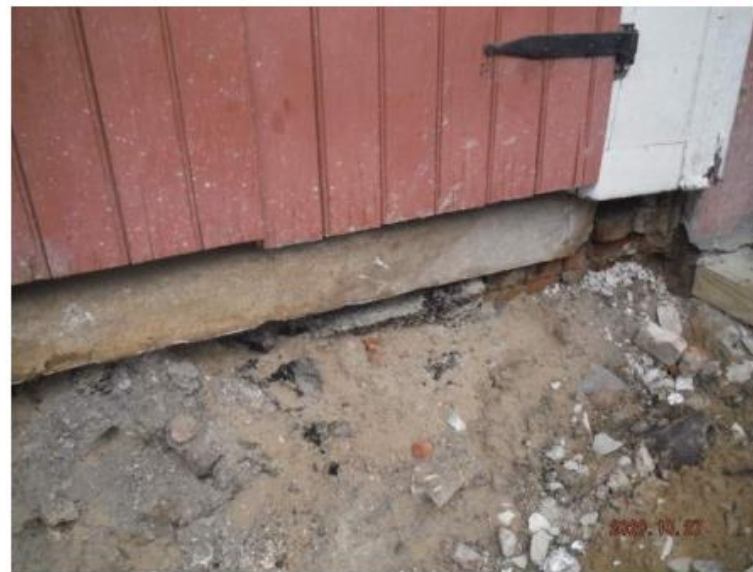
Photo 4: DAMAGED FOOTING.
