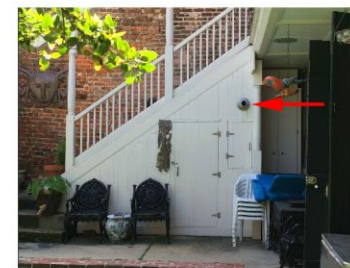
6 Underside of Stair Enclosed without Benefit of Permit Installation of Exhaust Vent without Benefit of Permit
