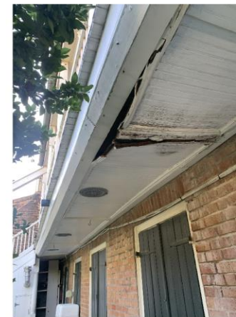
Inappropriate Ceiling & Trim-- To Be Removed
