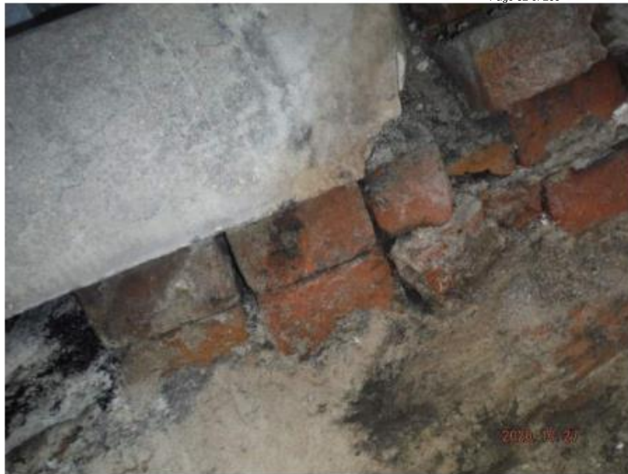
Photo 7: CLOSE UP OF DAMAGED AND DISPLACED BRICK IN FOOTING.
