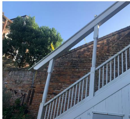
Inappropriate Lighting, Beam, & Columns To Be Removed Down To Handrail Scale: NTS
