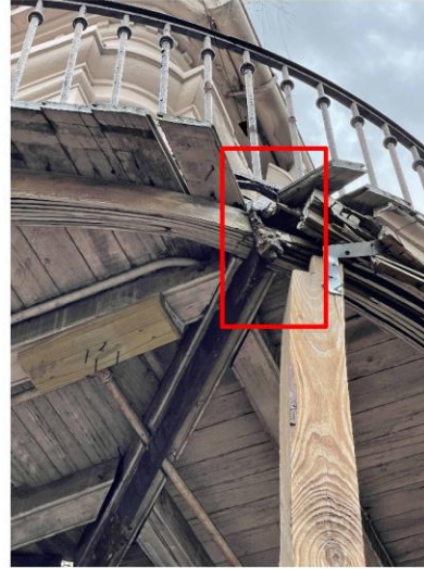
DAMAGED OUTRIGGER
