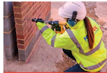
DryFix tie being power-driven into pilot hole
