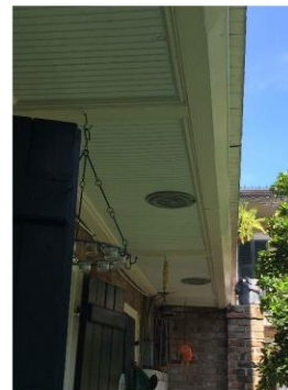
3 Inappropriate Balcony Underside Enclosure Recessed Lighting Installed without Benefit of Permit
