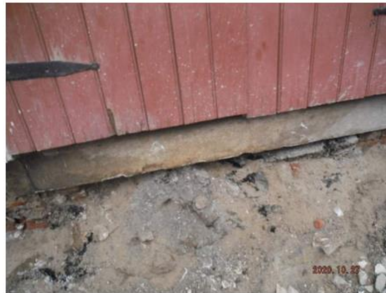
Photo 3: DAMAGED/MISSING FOOTING
