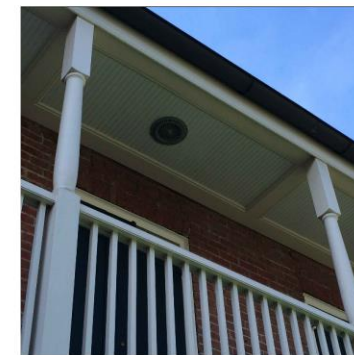
4 Inappropriate Coffered Balcony Ceiling Recessed Lighting Installed without Benefit of Permit
