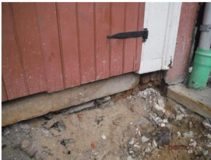
Photo 2: DAMAGED/MISSING FOOTING.
