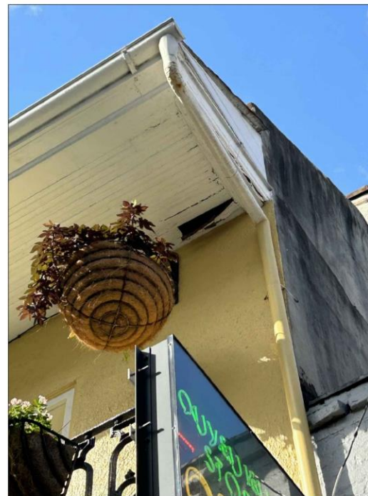
19 soffit repair
