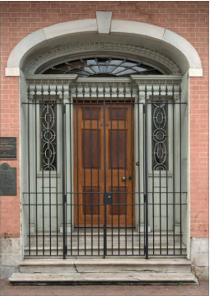
The security gate is sized to fit the opening and aligns with frames and muntins with a simple barrier grille and no decoration. The decorative fanlight transom remains visible.
