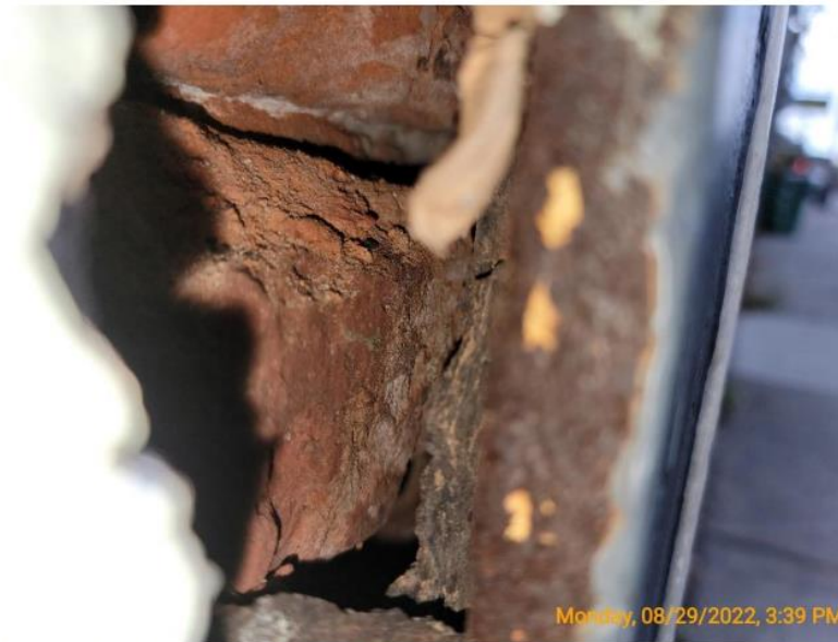
This is a limited view inside the wall cavity showing separation between the stucco cladding and the masonry wall.
