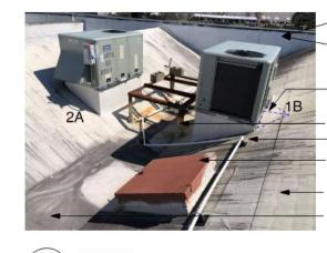
WALL BASE BID: New TPO 60 mil membrane in 2' horizontal layers secured to wall with continuous termination bars-fully adheared 150 MPH wind load based on manufacturers calculations and associated uplift pressures for this project.
