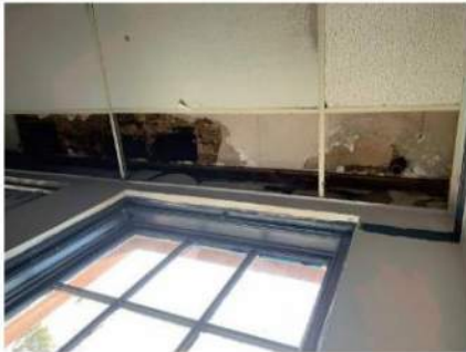
Water damage to ceiling D302
