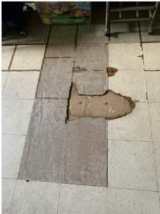
D 304 Water/termite damage to floors and baseboards
