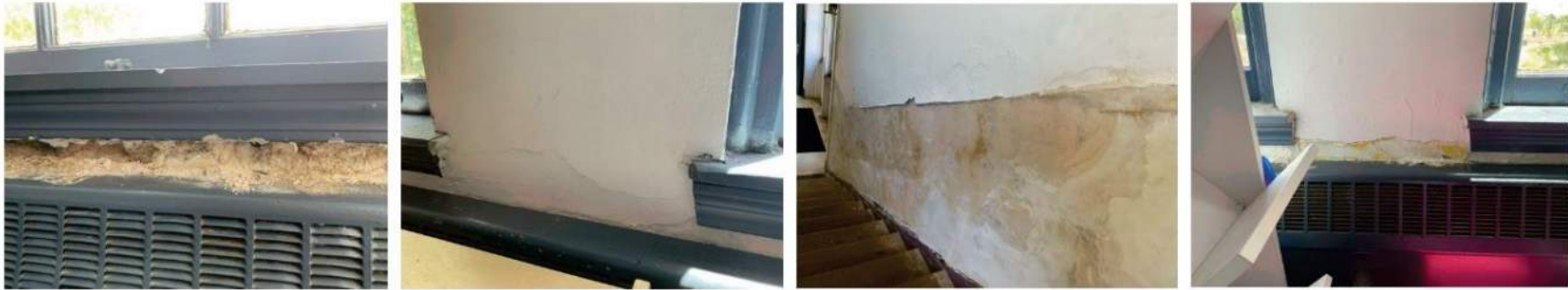
D200 and D300 Water Damage to Plaster
