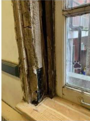
D 301 Water/termite damage to Window Sills and baseboards
