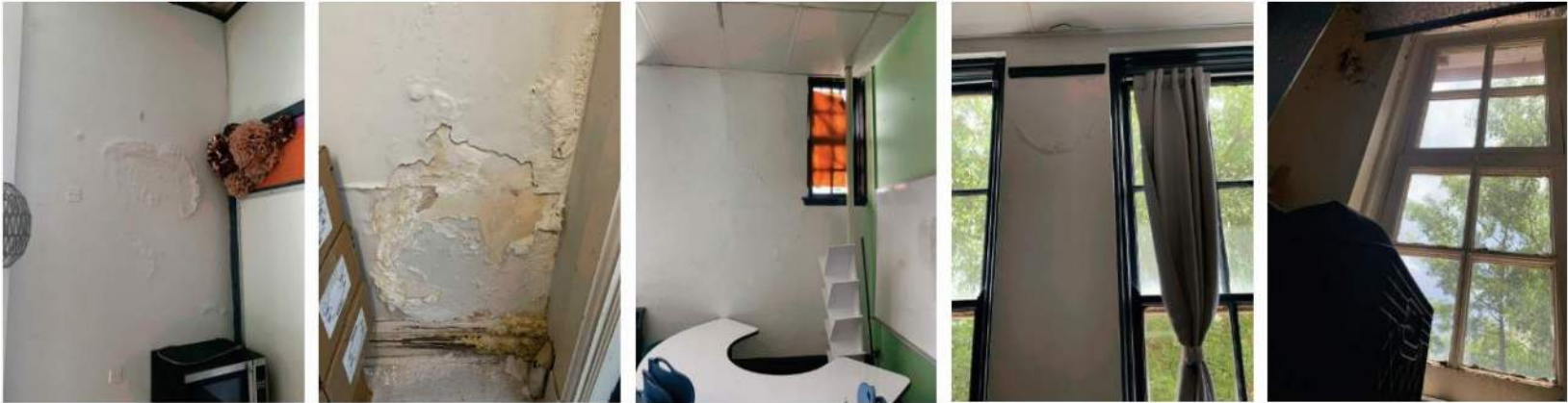
D200 and D300 Water Damage to Plaster
