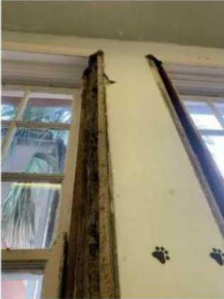
D 301 Water/termite damage to Window Sills and baseboards
