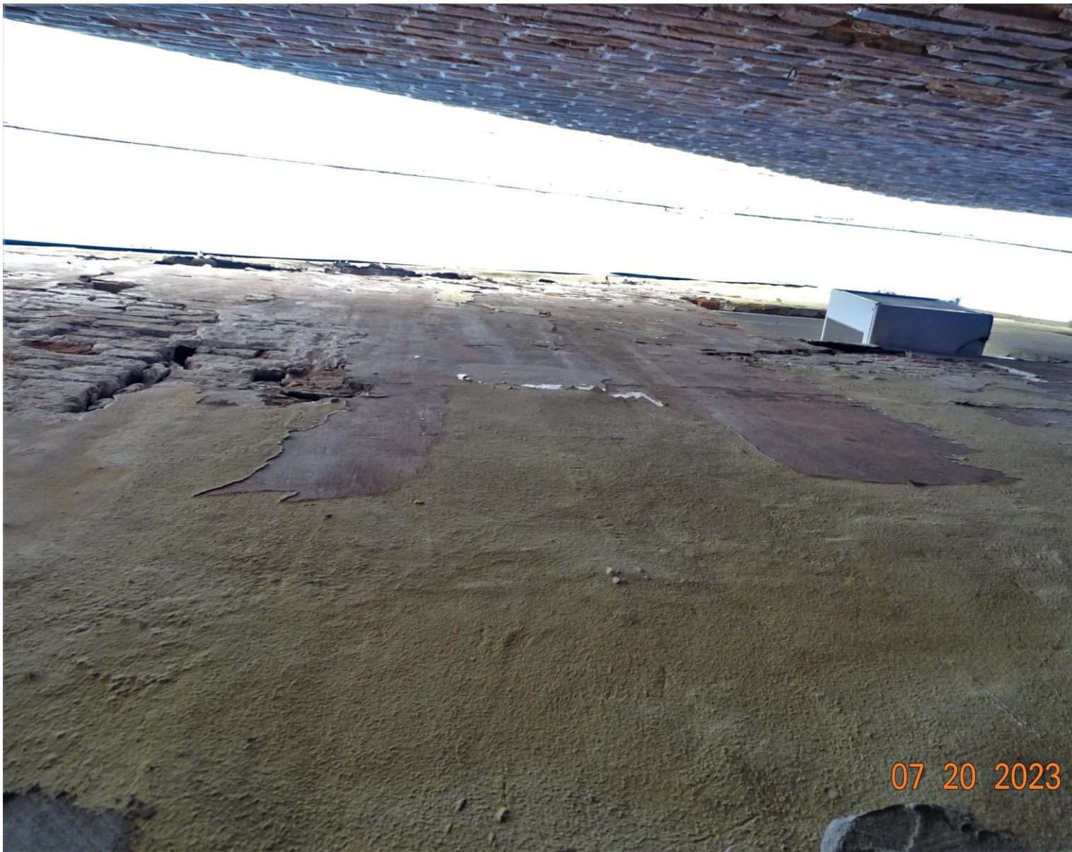
Dauphine elevation section with no thin-set mortar or mesh
