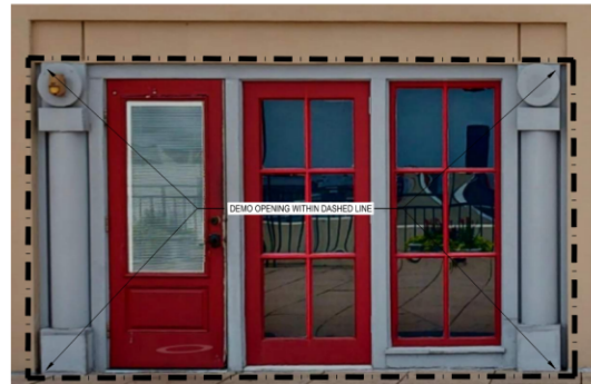
3 EXTERIOR DEMO MATERIAL LIMITS A3.06/ NO SCALE
