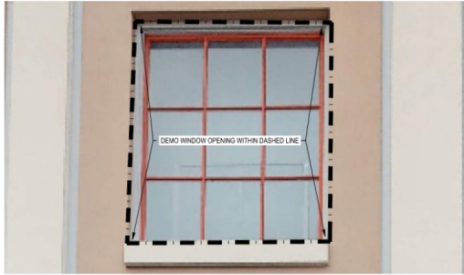
3 EXTERIOR DEMO MATERIAL LIMITS A2.00 NO SCALE
