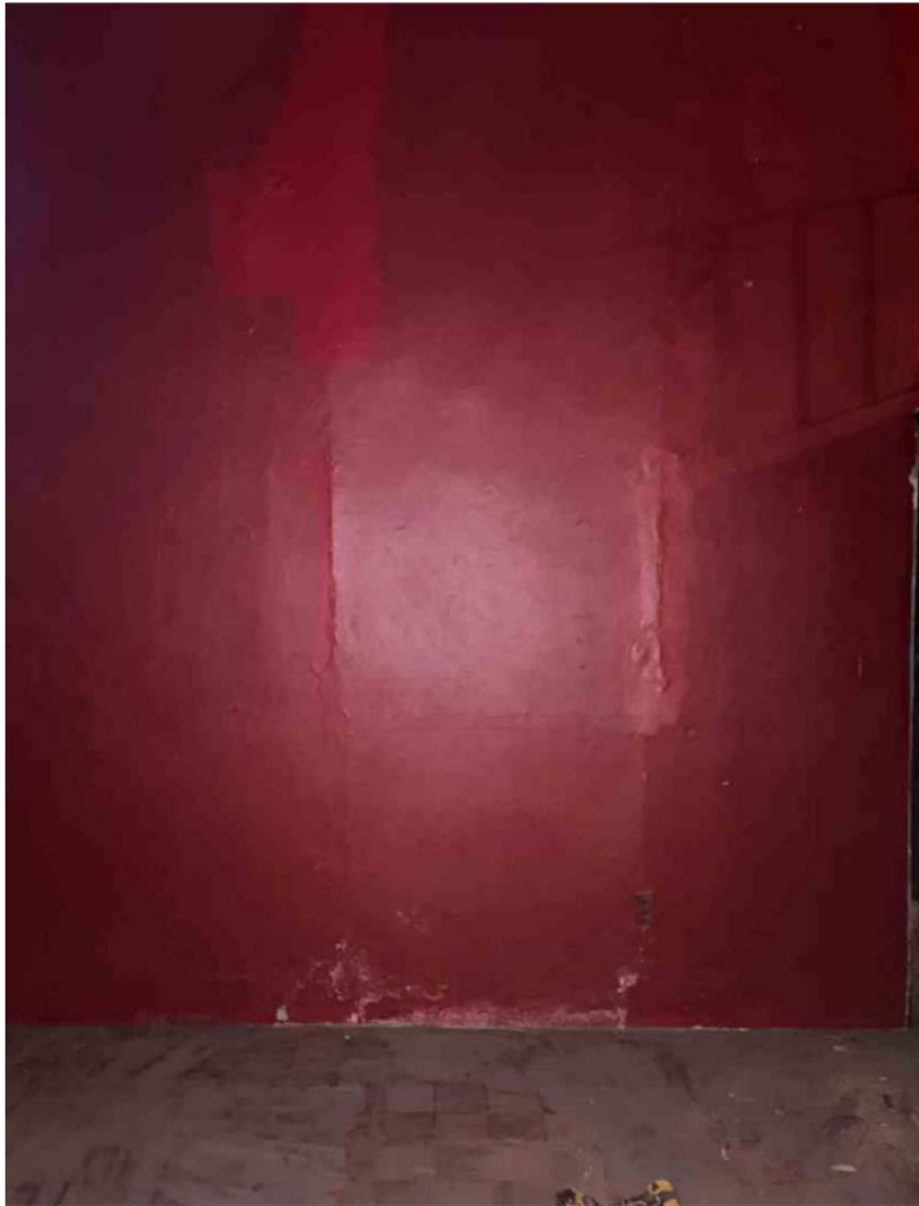
INTERIOR FRONT LEFT ROOM 1113 DAUPHINE - PLASTER CRACKING AT FORMER OPENING LOCATION (TO BE REUSED FOR NEW DOOR ASSEMBLY)
