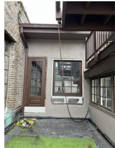
EXISTING DAMAGED WINDOW
