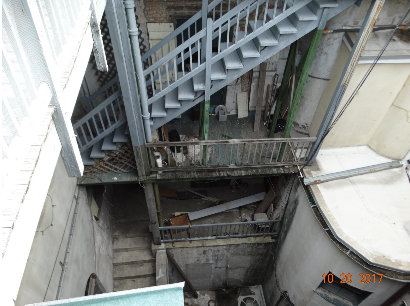
636-40 Royal – Courtyard Before Renovation
