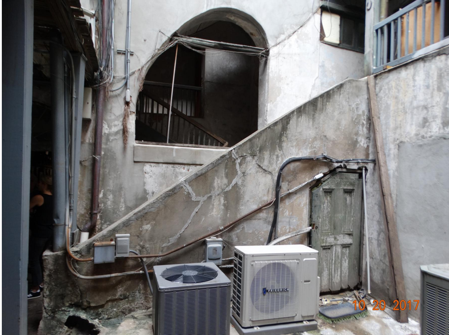
636-40 Royal – Courtyard Before Renovation
