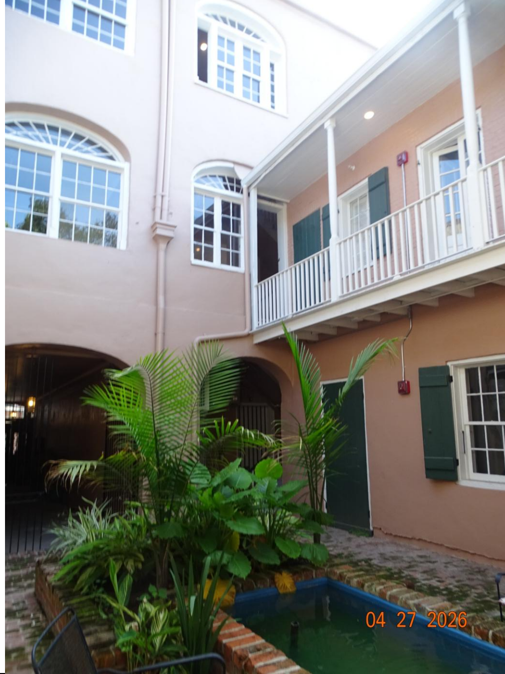
518 Governor Nicholls – After Renovation
