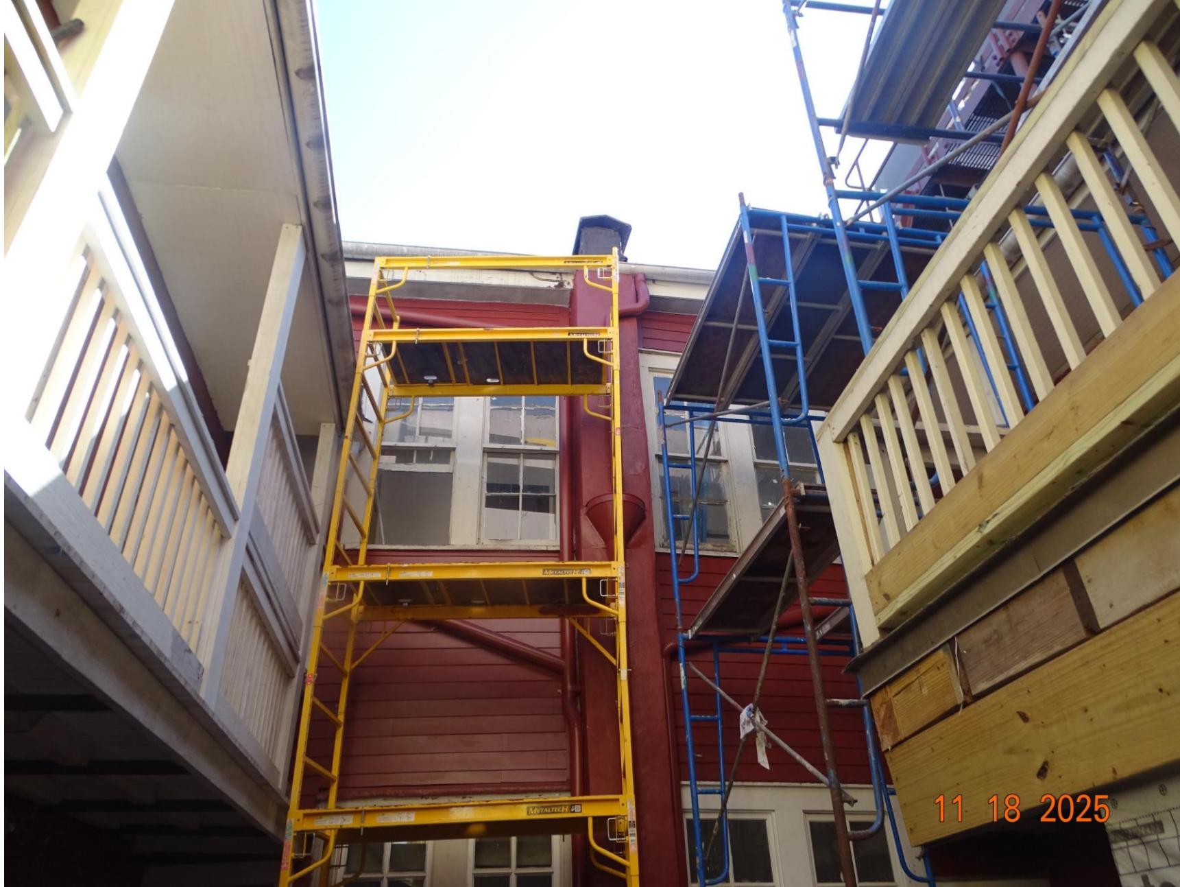
235-41 Bourbon – Courtyard Wall rebuilt and windows replaced
