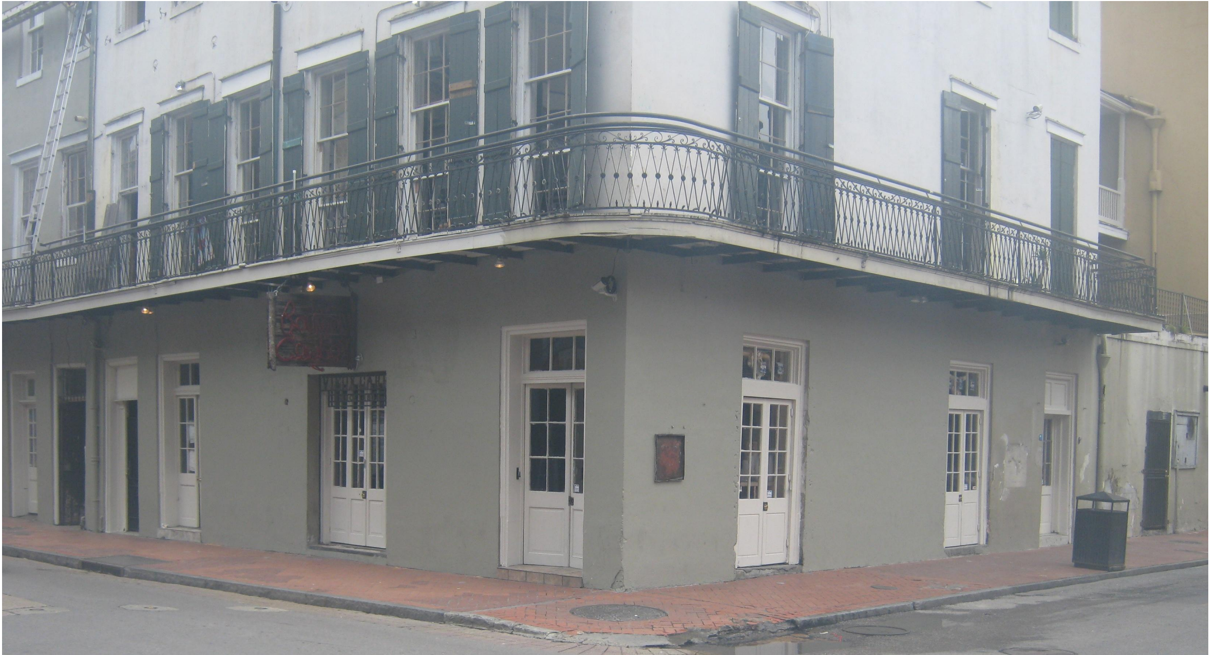
235-41 Bourbon – 2010 Repairs in Progress
