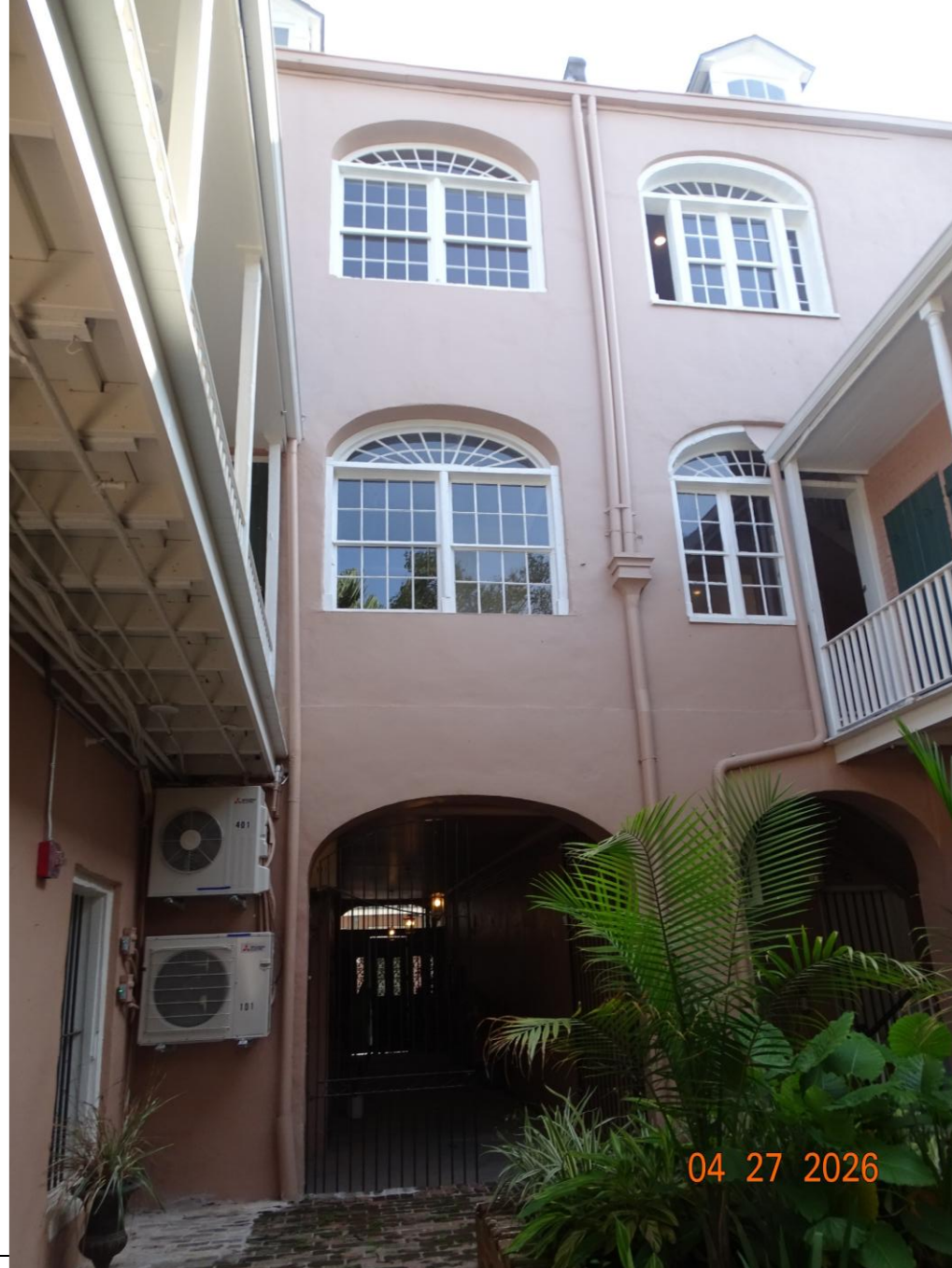
518 Governor Nicholls – After Renovation
