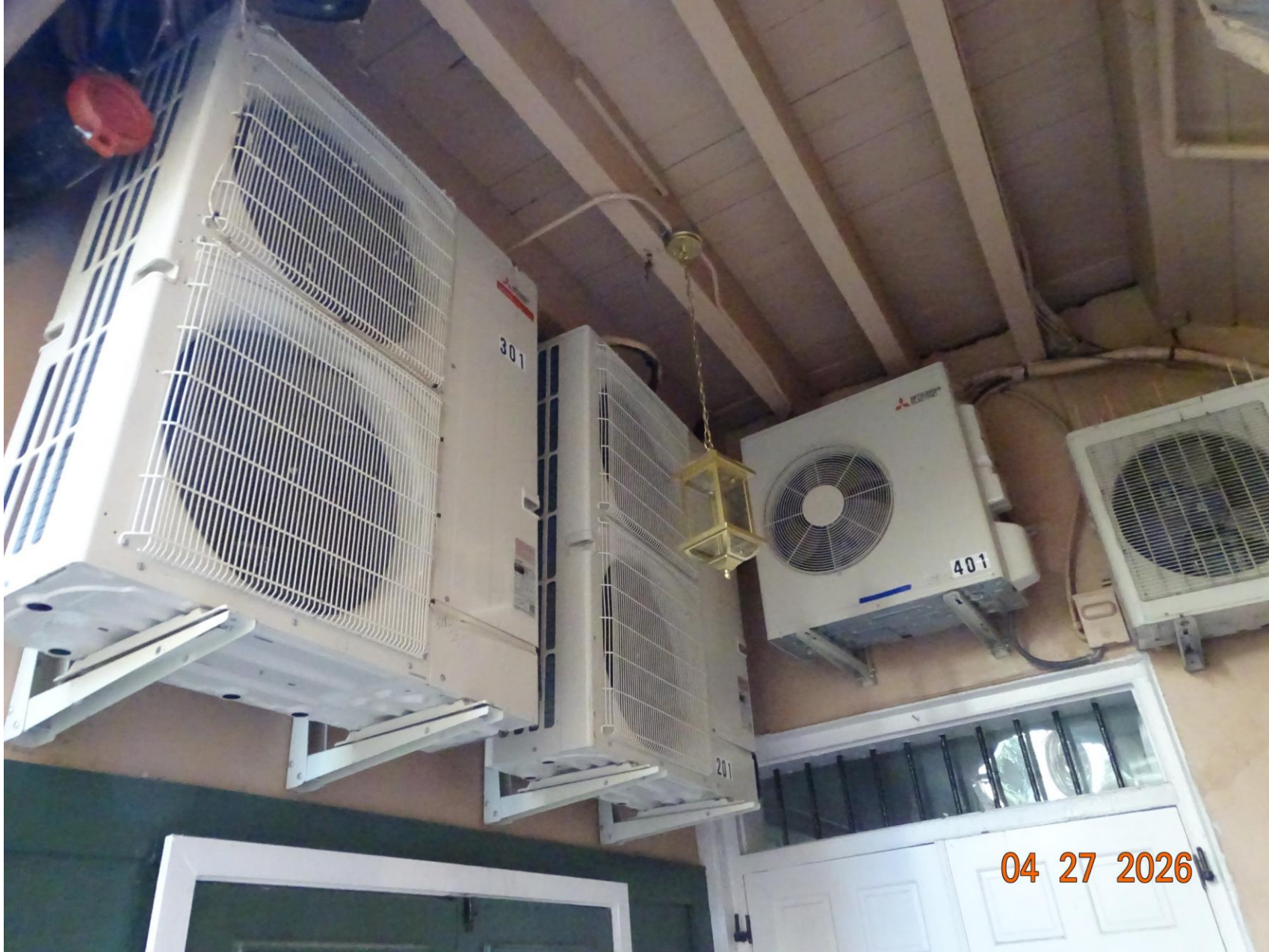
518 Governor Nicholls – After Renovation
