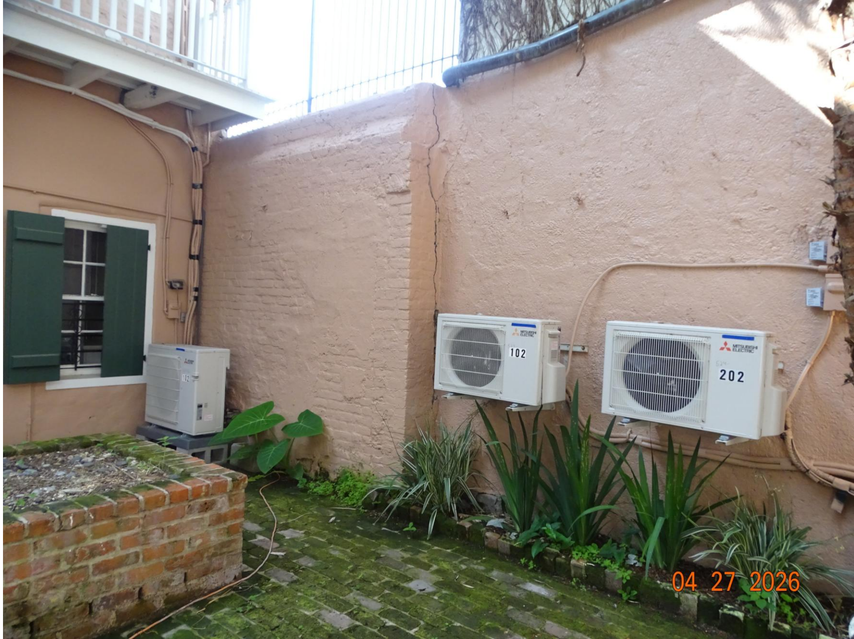
518 Governor Nicholls – After Renovation
