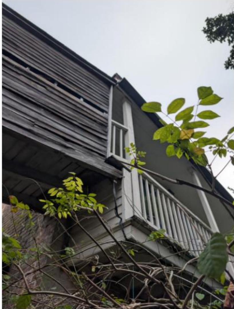
Multiple Sanborns show consistence in location of catwalk. Drawn with dotted line implying an open air structure.
