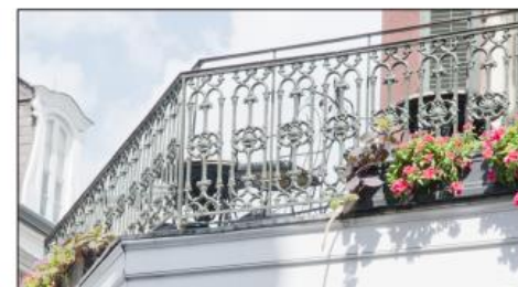
A discrete, higher secondary safety rail has been installed behind the cast iron balustrade to meet building code requirements. An alternative would be to raise the historic balustrade to the required height.
