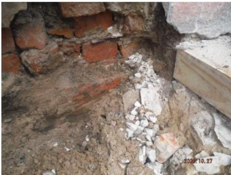
Photo 5: CLOSE UP OF DAMAGED BRICK OF FORMER FOOTING.
