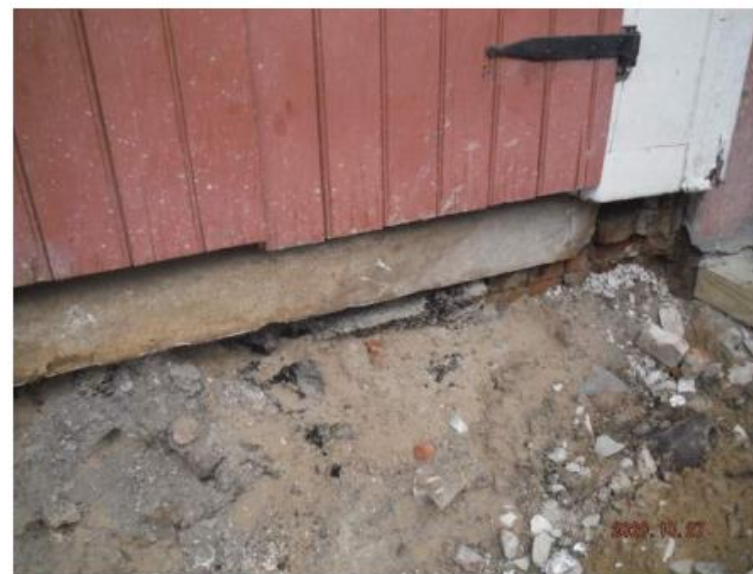
Photo 4: DAMAGED FOOTING.
