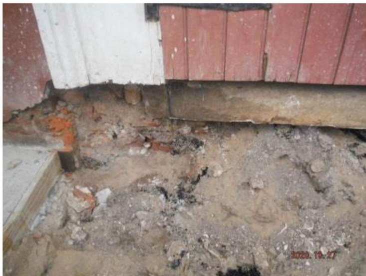
Photo 1: DAMAGED FOOTING
