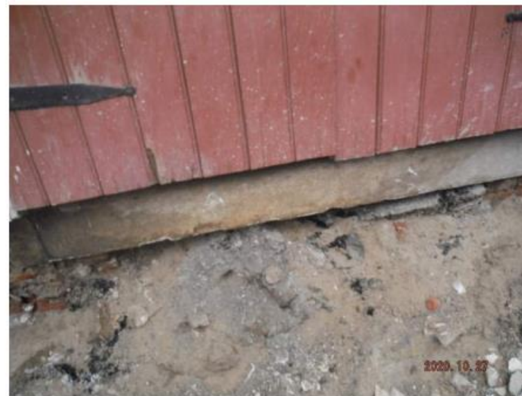
Photo 3: DAMAGED/MISSING FOOTING
