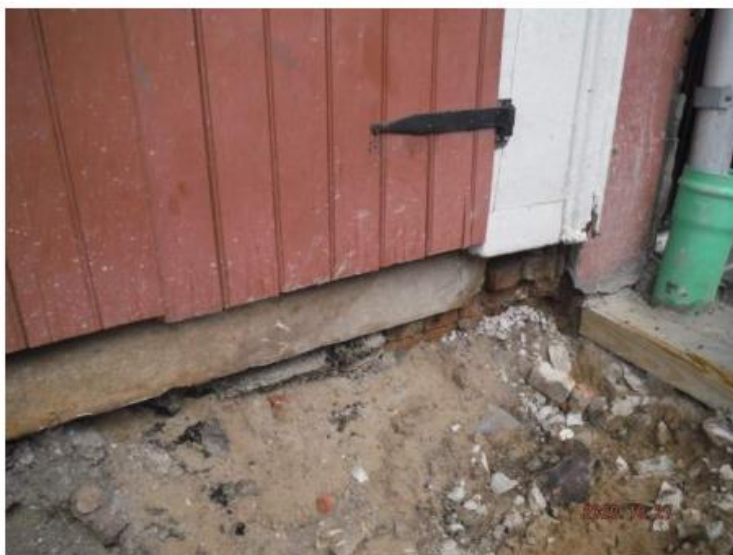
Photo 2: DAMAGED/MISSING FOOTING.
