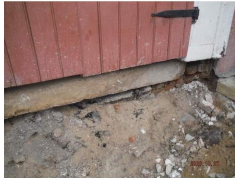
Photo 4: DAMAGED FOOTING.
