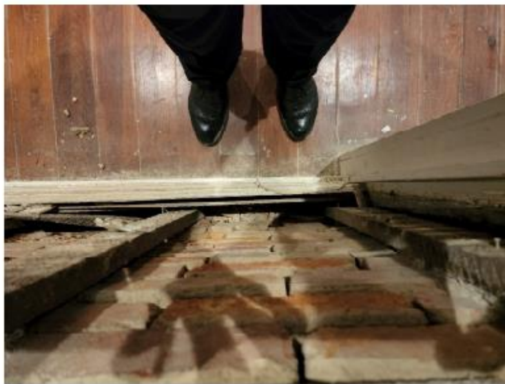
Photo 2: Inside face of front wall. Note lack of mortar.
