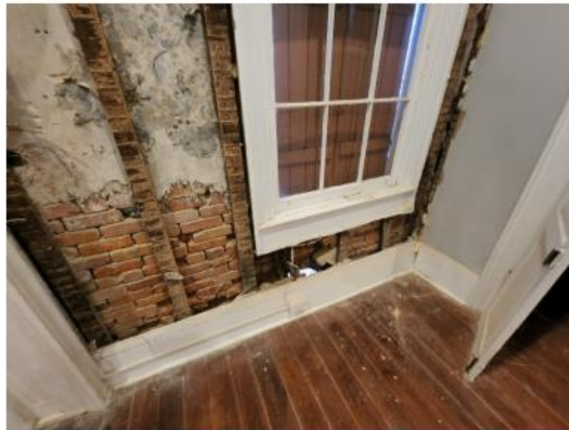
Photo 4: Note the area of collapsed brick below window.
