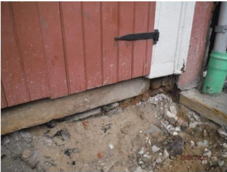
Photo 2: DAMAGED/MISSING FOOTING.
