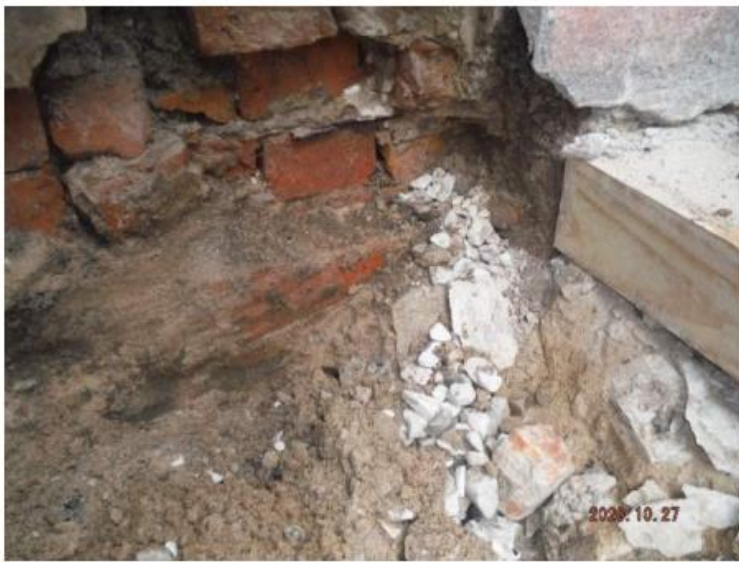
Photo 5: CLOSE UP OF DAMAGED BRICK OF FORMER FOOTING.
