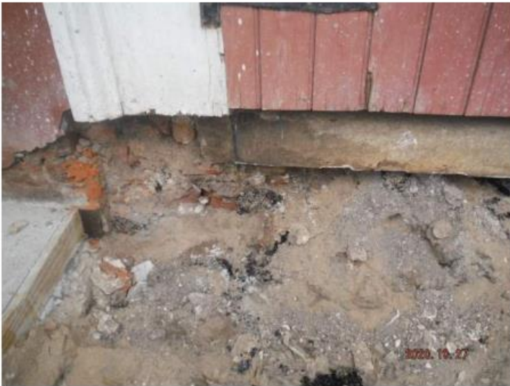
Photo 1: DAMAGED FOOTING
