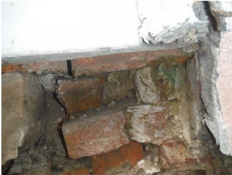
Photo 6: CLOSE UP OF DMAGED BRICK IN FORMER FOOTING.
