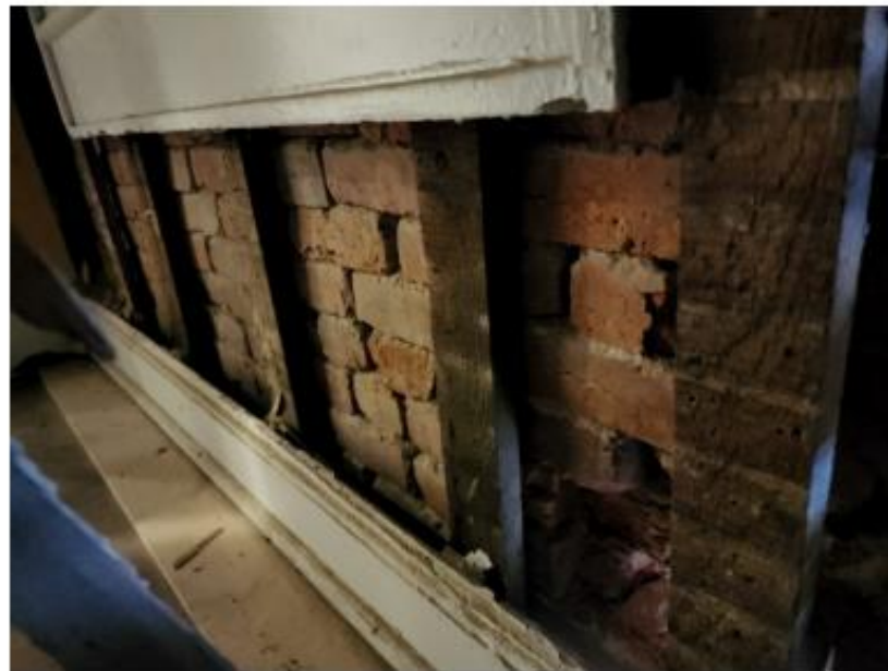
Photo 3: Inside face of wall, no mortar in joints.
