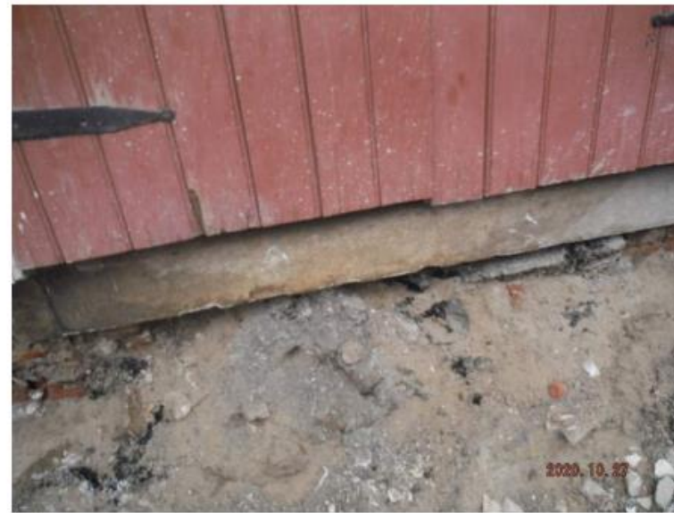
Photo 3: DAMAGED/MISSING FOOTING
