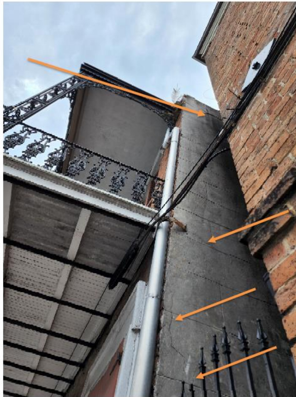
Photo 8: Cracks at side wall.
