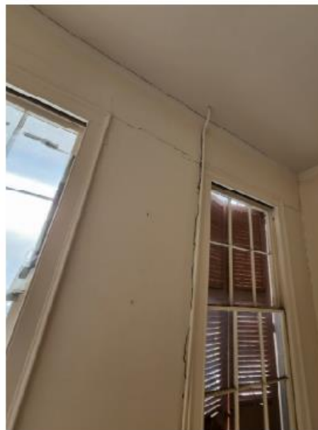
Photo 6: Cracking in Front wall at second level.
