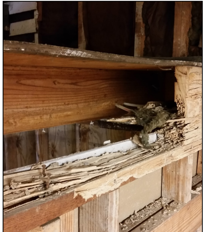
Figure 53. Termite damage above the mechanic's office that had to be repaired prior to renovations.
