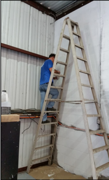
Figure 54. LJ Kabel applying a coat of primer paint to the walls of the automotive maintenance shop.
