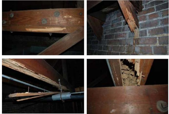
**Figure 32.** Extensive structural damage to attic area of the Cita Dennis Hubbell Branch of the New Orleans Public Library remaining from a termite infestation remediated in 2005.
