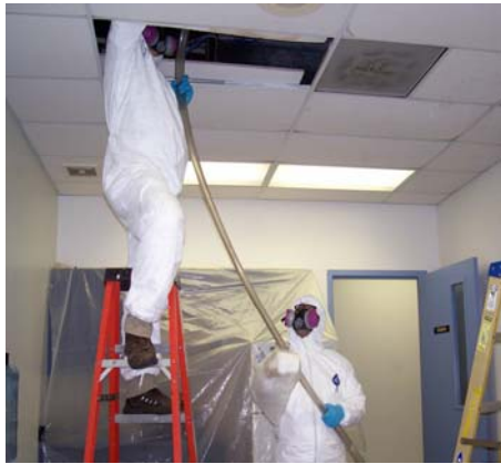
Figure 1. LJ Kabel and Jimmy Jesse clean-up and repair the Biolab building.
