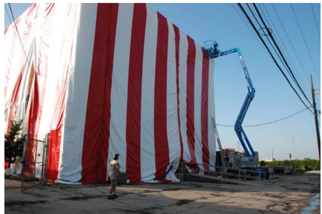
Figure 5. Fumigation of the public works building at 838 S. Genois Street.
