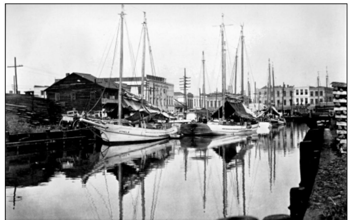
The turning basin of the New Orleans (New Basin) Canal terminated at South Rampart Street between Julia and DeLord (Howard) Streets. The townhouses on the right were situated on South Rampart Street. Although the photograph shows several schooners, companies transported goods on the canal with small steamboats and barges pulled by mules. [State Library of Louisiana 1929]
