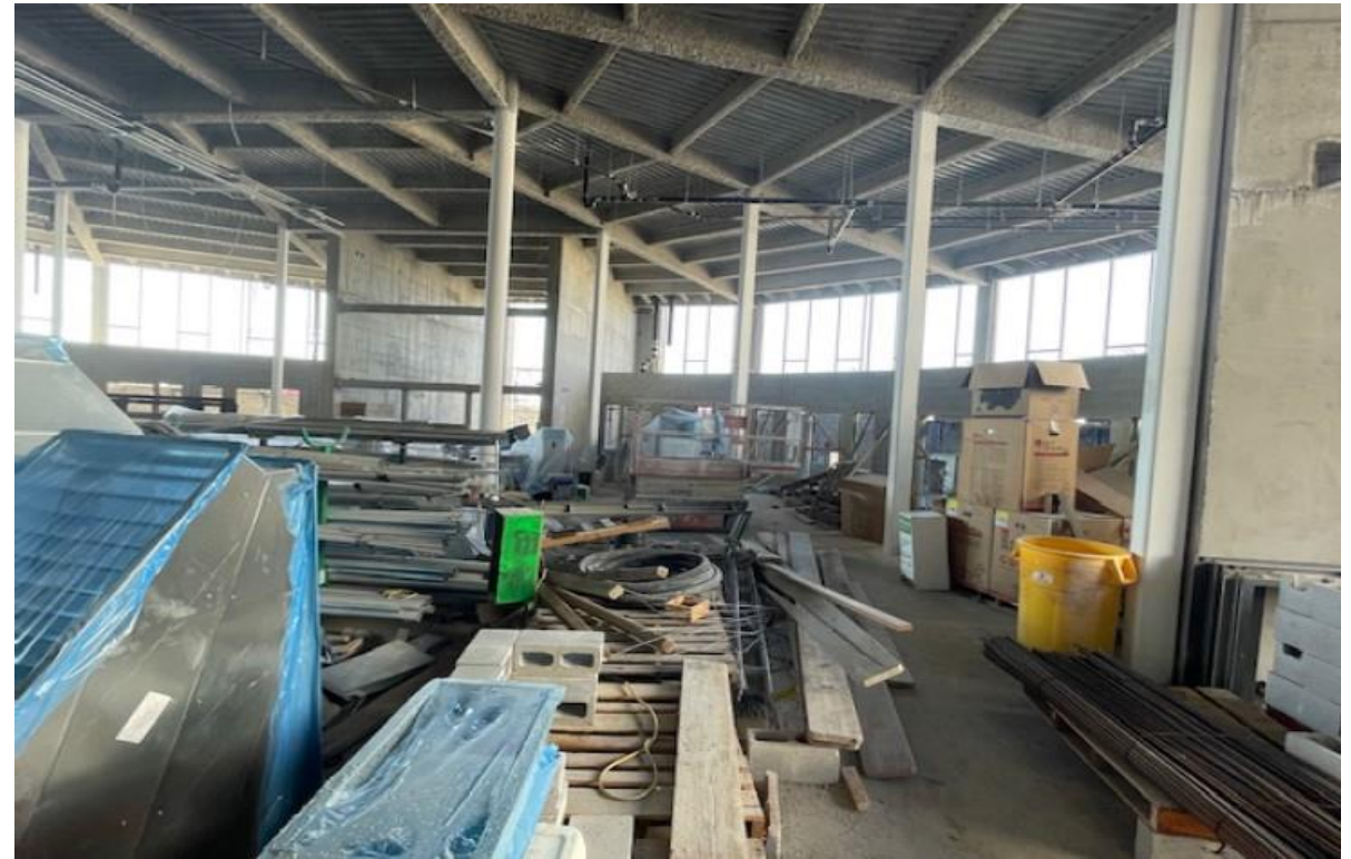
OJC Medical Services Building
