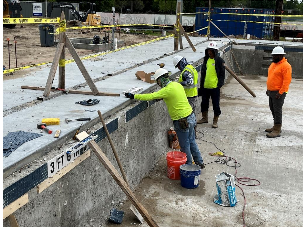
M.X. Jeff Pool Renovations
