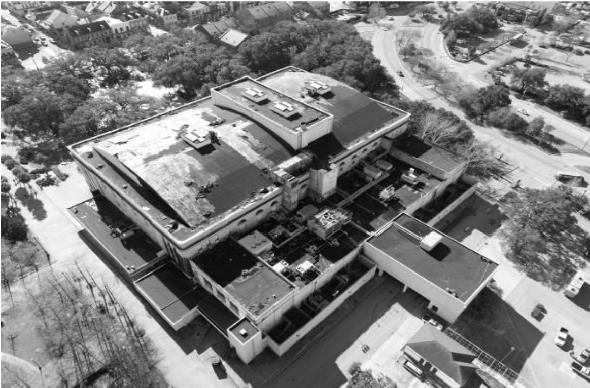
Municipal Auditorium Exterior Repairs
