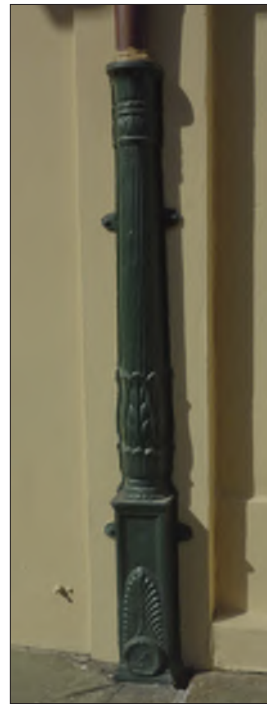
A decorative cast iron boot should be retained.
