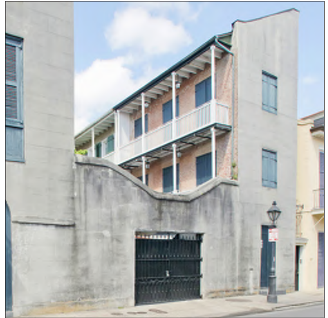
Some service buildings are partially hidden from view by a courtyard wall. In this case, the outbuilding is located along the rear property line of the principal building.
