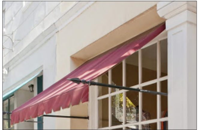
This sloped awning has open sides and decorative metal rods providing support.
