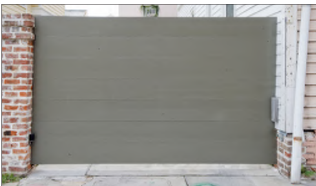
This automatic gate provides vehicular access into the courtyard. The door sensor is discretely located near the bottom of the brick pier on the left.
