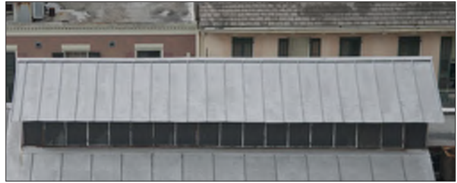
This roof monitor is located along the roof ridge and includes a continuous row of windows.
