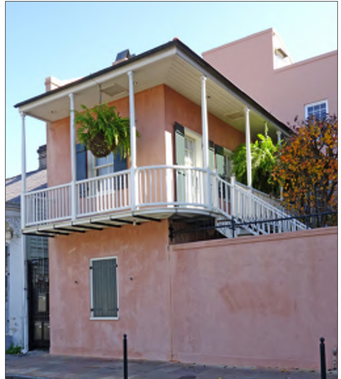
This secondary structure was constructed in 1998 at the rear of the courtyard using materials and simplified details that are compatible to the main house.
