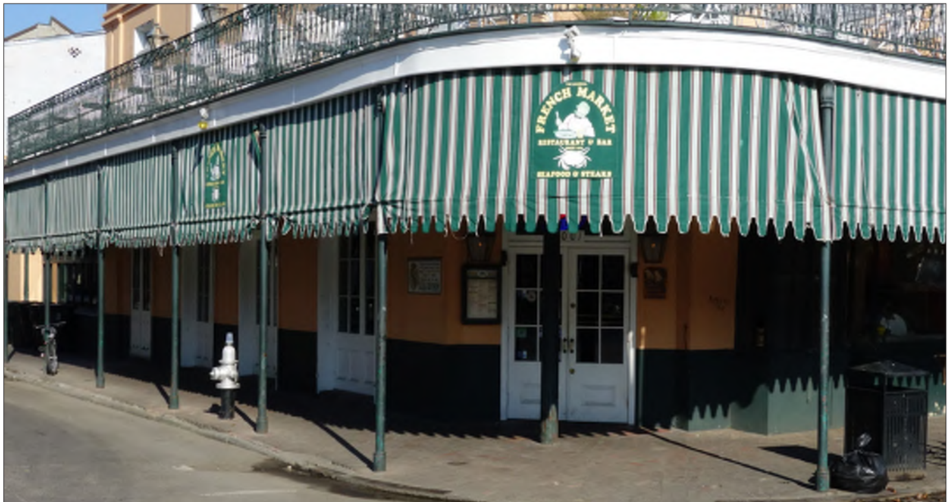
These drop awnings are located between each of the building's bays, providing a unifying element for the storefront and providing shade in the morning sun. The business name on the corner is of a larger scale, appropriate for the vehicular traffic along Decatur Street.
