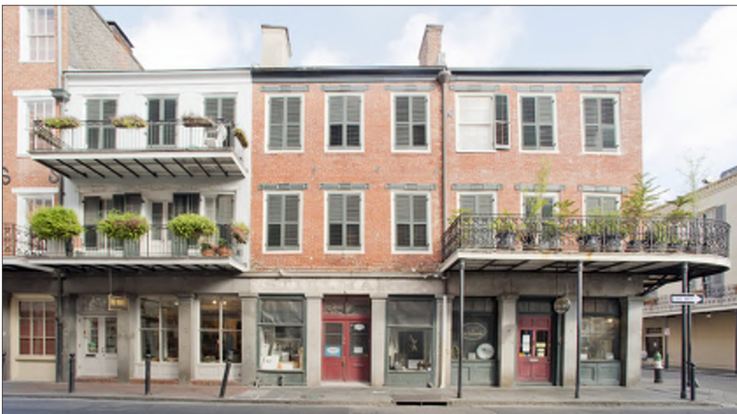
It appears that these three buildings were constructed at the same time. They share several characteristics and architectural features. The center building does not include a balcony or gallery, although evidence at the wall surface suggests a gallery or balcony may have existed previously. With appropriate documentation, obtaining VVC approval for the reconstruction of the gallery or balcony might be possible.
