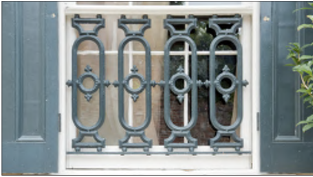
A cast iron decorative railing, sometimes found at a window, may include a repetitive pattern of detailed components.
