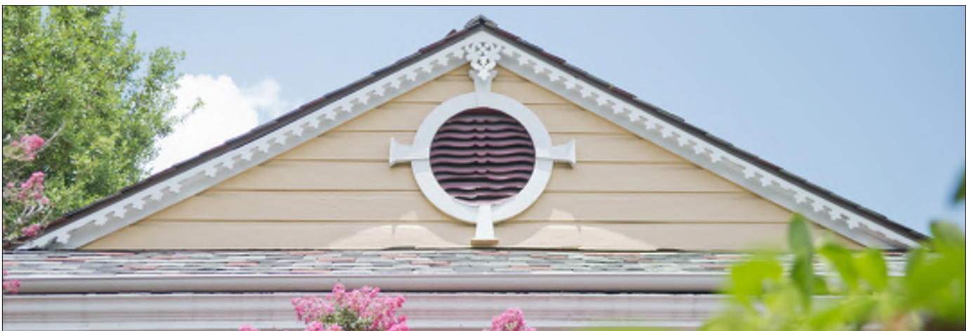
Gable ends of shotgun residences often include decorative woodwork. This example has a decorative rake board, drop lap siding and a central, bulls-eye louver with profiled slats. (Gable-end louvers should be covered in the event of a storm to prevent roof uplift. Refer to Storm Preparedness, page 05-10.)
