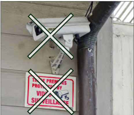
The installation of a large-scale box ("shoebox") camera and/or supplemental signage is not allowed by the VCC.
