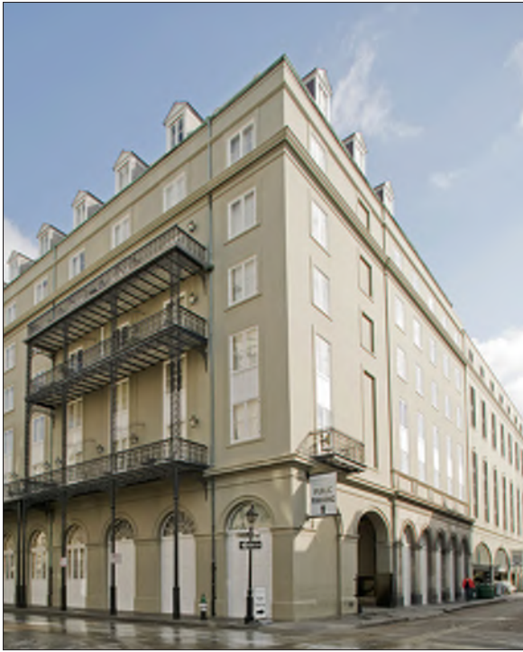
A first floor remnant of the old St. Louis Hotel remains to the right. In 1960, a larger hotel was constructed, incorporating the remnant, with compatible arched ground floor openings and storefront cornice.
