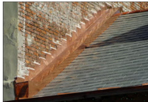
Newly installed, stepped copper flashing is located along the juncture of the parapet with the adjacent wall.
