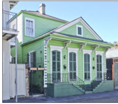
A camelback addition typically is found on a wood-framed shotgun single or double.
