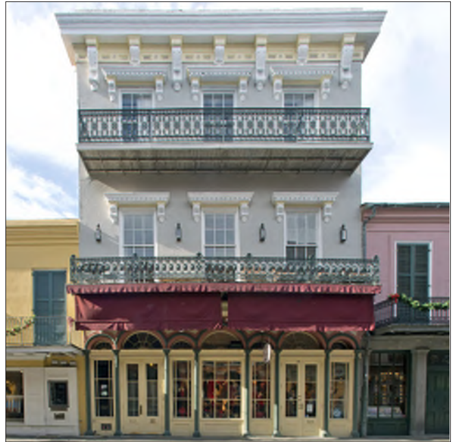
The heavy, bracketed building cornice, decorative window lintels and arched masonry openings at the ground floor are typical of the Italianate style.
