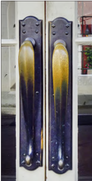
The bronze door hardware complements the style of the building.
