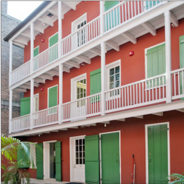
A balcony is used for circulation in an outbuilding. This example includes a 2-level, covered balcony providing access to each of the upper level rooms.
