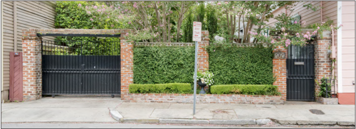
This brick wall conceals a garden beyond and includes access gates supported by brick piers for vehicles and pedestrians. A brick planter with shrubs and carefully maintained wall plantings is located between the gates, providing visual interest along the streetscape.
