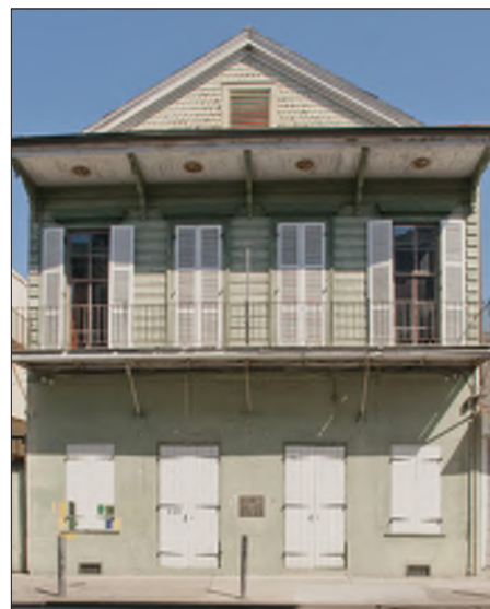
Determining the original type and style of a building can be challenging. The ground floor of this example has many of the characteristics of a Creole cottage, while the second floor addition has features of an Italianate shotgun double.
