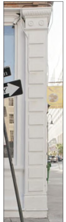
Cast Iron Pilaster With Applied Quoins
