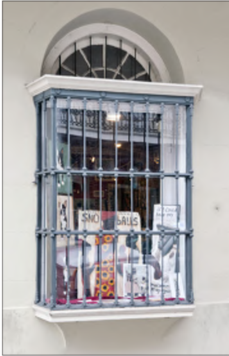
The decorative metal security grille at this projecting display window is historic and an integral part of the original design.
