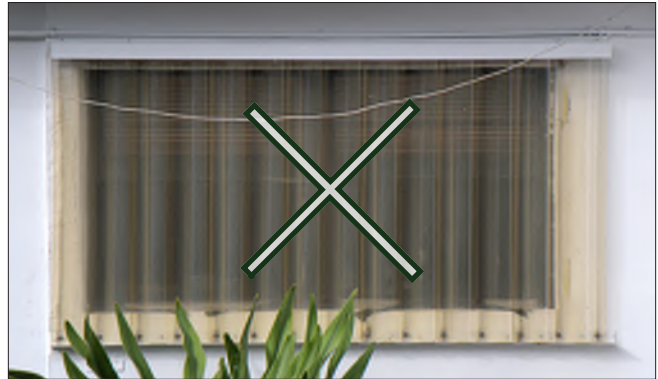
Permanently attached plastic storm protection panels are not appropriate in the Vieux Carré.
