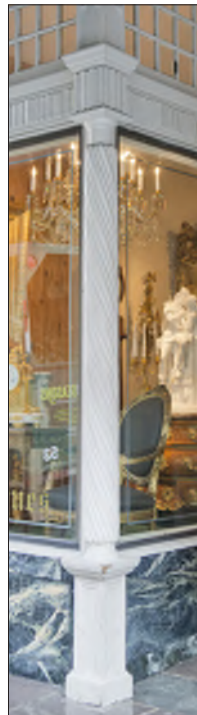
Decorative Cast Iron Window Support
