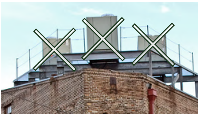
The visibility of mechanical equipment should be minimized and located to least disrupt the appearance of the historic building, streetscape and District.
