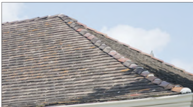
Historically, terra cotta tiles were available in a variety of shapes, including plain rectangular tiles, as shown above, similar in form to slate.
