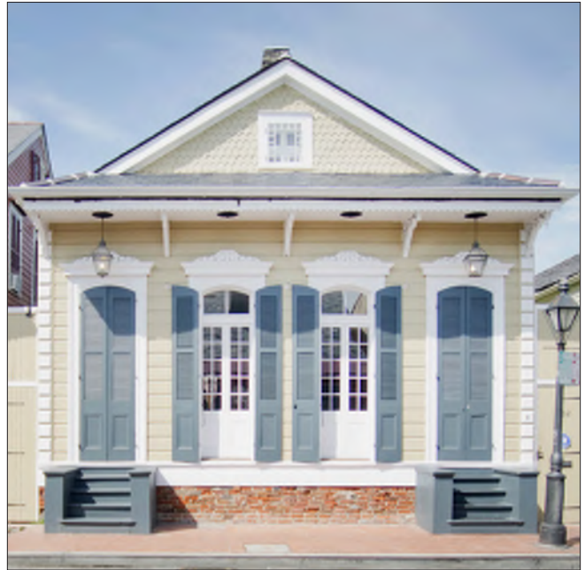
A shotgun double is typically 4-bays wide and includes paired central windows or French doors flanked by entrance doors. They frequently are converted into a single residence, although their separate entrance stoops must be maintained.
