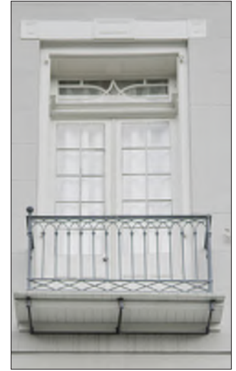
A "basket" or "box" balcony may be found on upper floors of pre-1835 buildings.
