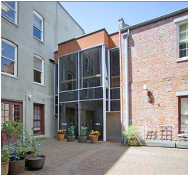
A 1975 addition with modern materials links the main and service buildings in this courtyard.
