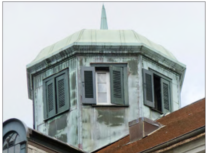
While a roof monitor is generally rectangular and located along the roof ridge, a cupola tends to be round, square or octagonal, as in this example.
