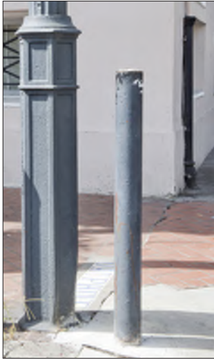
A pipe bollard has been installed to protect the cast iron column from impact.
