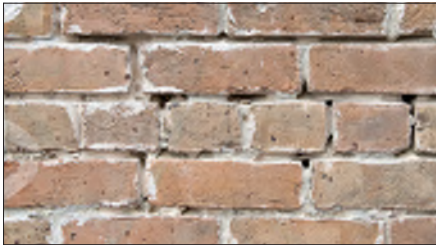
Local 19th Century Brick – A soft, fired-clay, fairly regularly-shaped building component; locally known as lake or mud brick; often with color and surface variations; used primarily in walls, piers, foundations and exterior paving.
