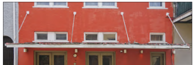
This canopy is suspended from above by cables and is located between the transom windows and doors below.
