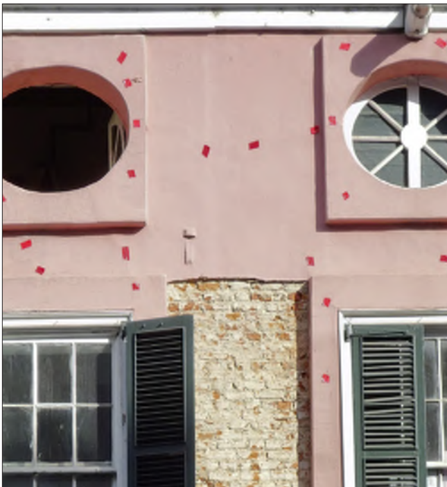
The stucco wall is in the process of repair. The loose stucco between the windows has been removed to the brick substrate to allow the new stucco to be installed. Red tape marks the locations of cracks to be repaired.
