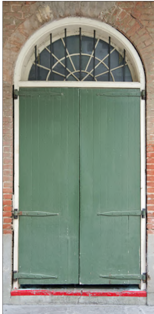
This opening is secured using traditional materials. The half-round window has inset metal bars and the solid wood shutters cover the entry.
