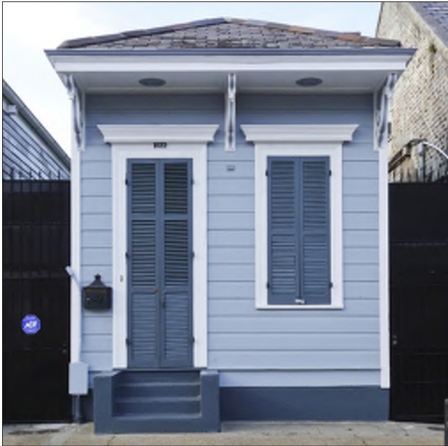
A shotgun single is 2- or 3-bays wide with rooms extending toward the rear of the property, fitting well on a long, narrow lot.
