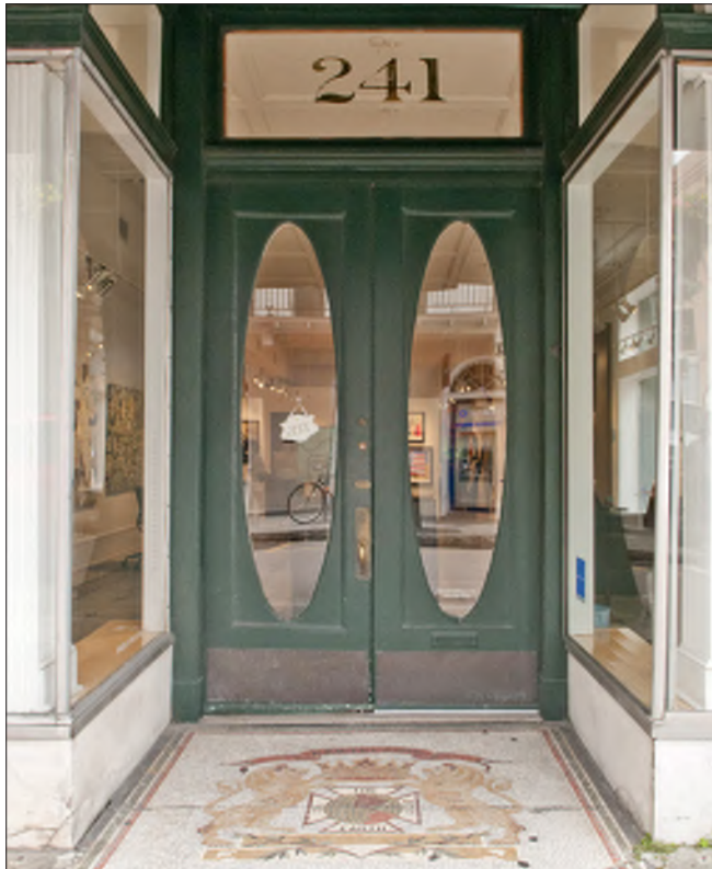
The oval lights, or windows, in this paired entrance door are unusual for the Vieux Carré and likely date to the early-20th century. Note the large transom window with street number above and the decorative tile alcove flooring below.
