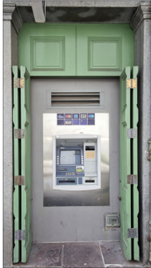
The shutters have been modified for the installation of this ATM between the granite piers. The shutters can be closed to provide additional security and conceal the ATM from view.
