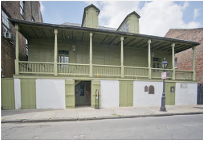
The 1788 Madame John's Legacy House, a National Historic Landmark, is one of the oldest documented buildings in the Vieux Carré and is typical of French colonial houses.
