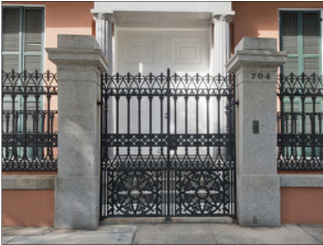
This elaborate cast iron entrance gate is supported by granite piers. It is of similar design to the cast iron fence mounted above the stucco chain wall which includes a granite cap.
