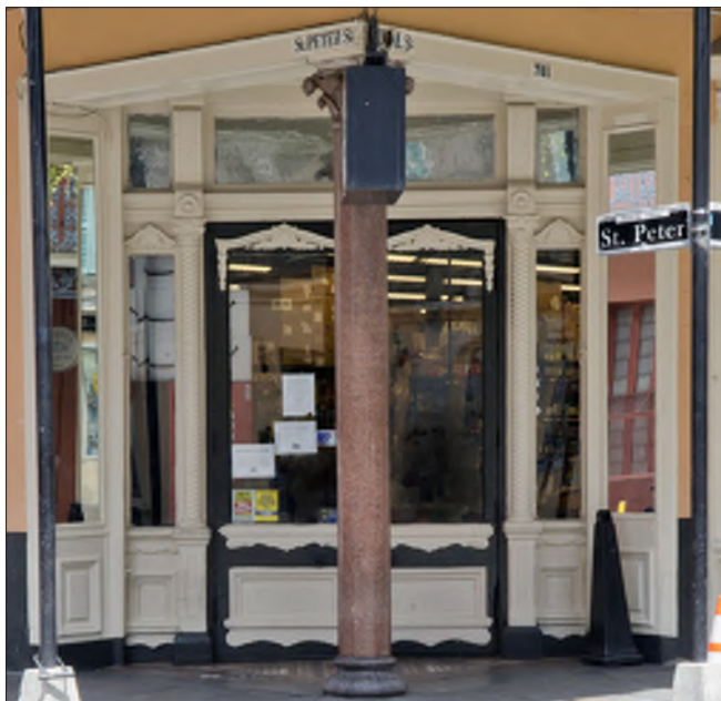
This paired, corner entrance door includes sidelights and a transom above. Note the granite corner support column.
