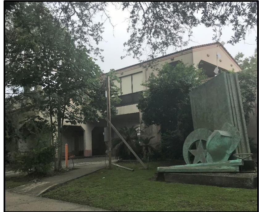
Figure 6: Front Façade of the existing NOFD Headquarters
